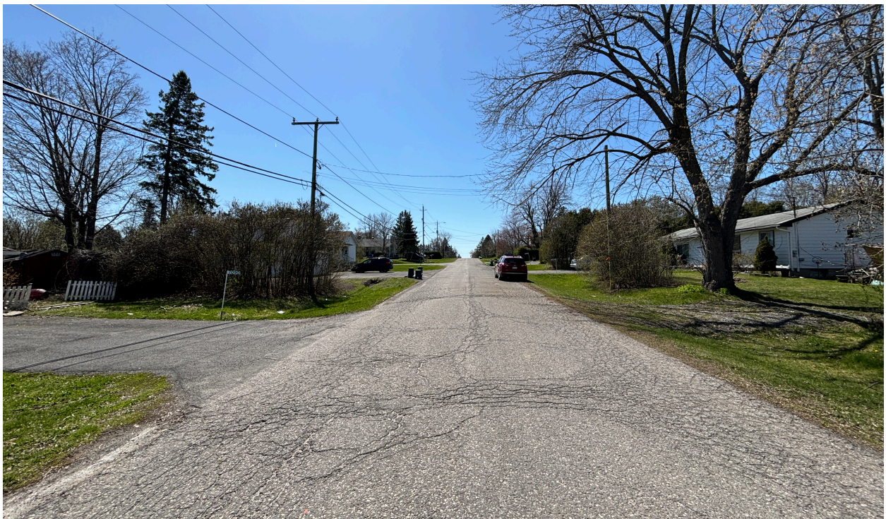
Figure 7: Marco Street, looking west
