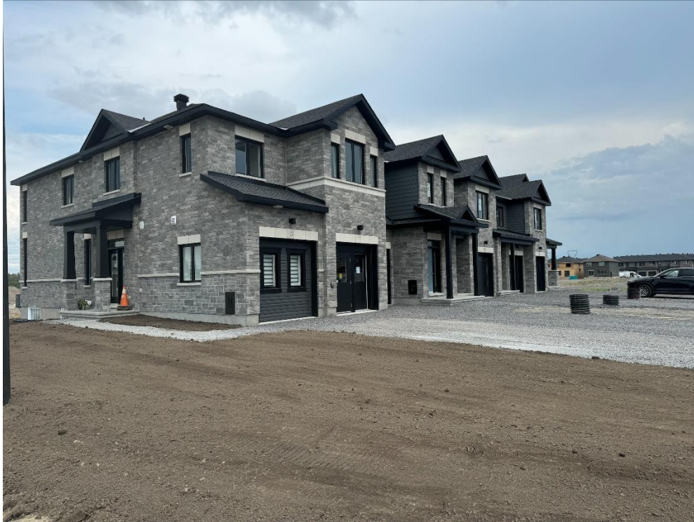
Photo of 1126 Cope Road (June 21, 2024)
