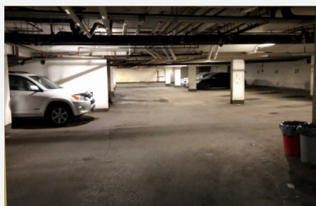
McAuley Place, 450 Laurier Avenue: Structural Rehabilitation to the Underground Parking Garage
