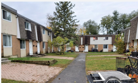
Michele Heights: Exterior Site Renewal to 132 Homes
