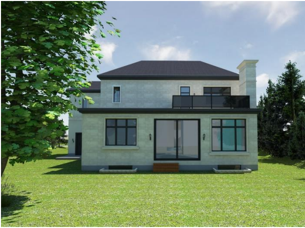
Figure 8: West elevation – rear façade
