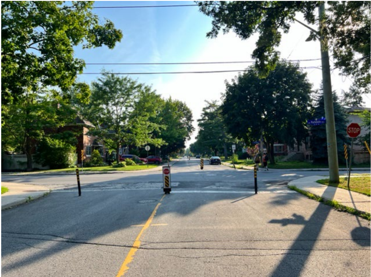
Figure 1 - Image of an All Way Stop Control (AWSC) flexible stake sign installation
