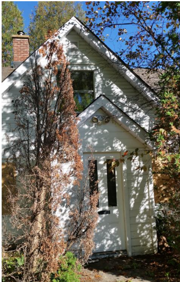
Photo showing the condition of the house before the development in 2015
