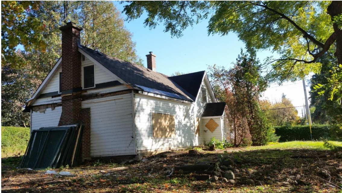
Photo showing the condition of the house before the development in 2015
