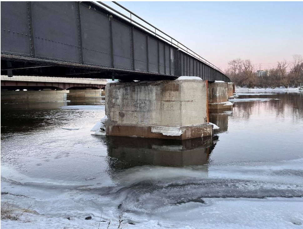
Photos of the bridge looking east
