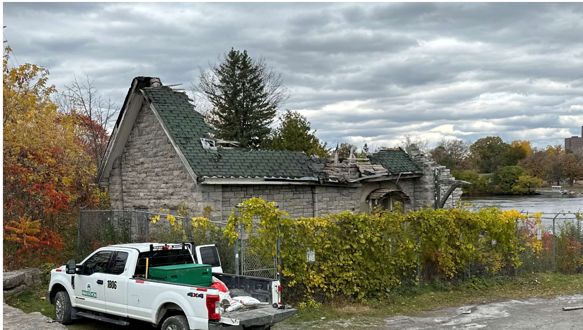
i View of Existing Pumphouse Ruin - source CSW
