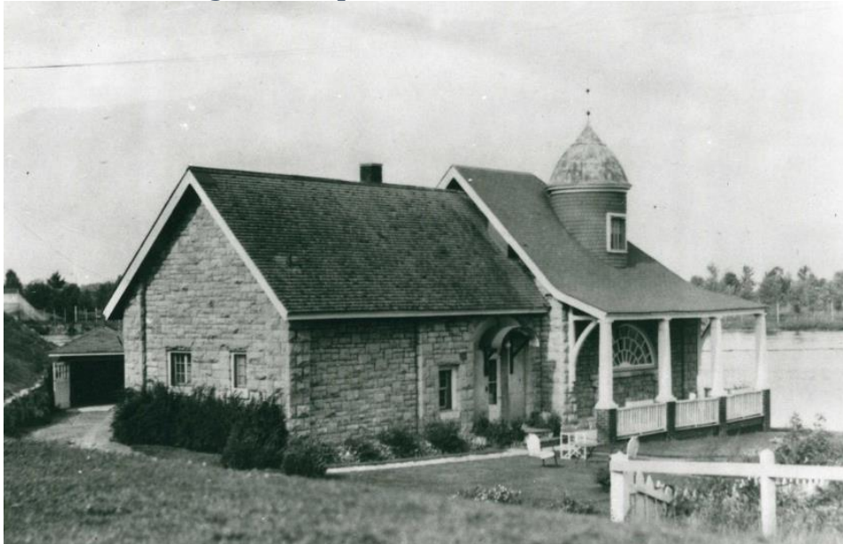
Figure 1: Hintonburg pumping station, 1928
