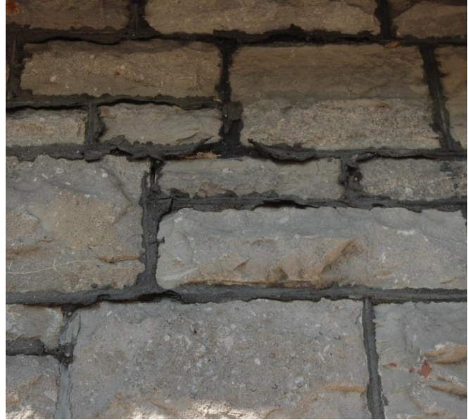
Figure 17: Portland cement repointing on south wall [JCAL 2021]
