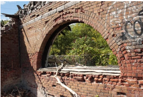
Figure 9: North window arch [JCAL 2021]
