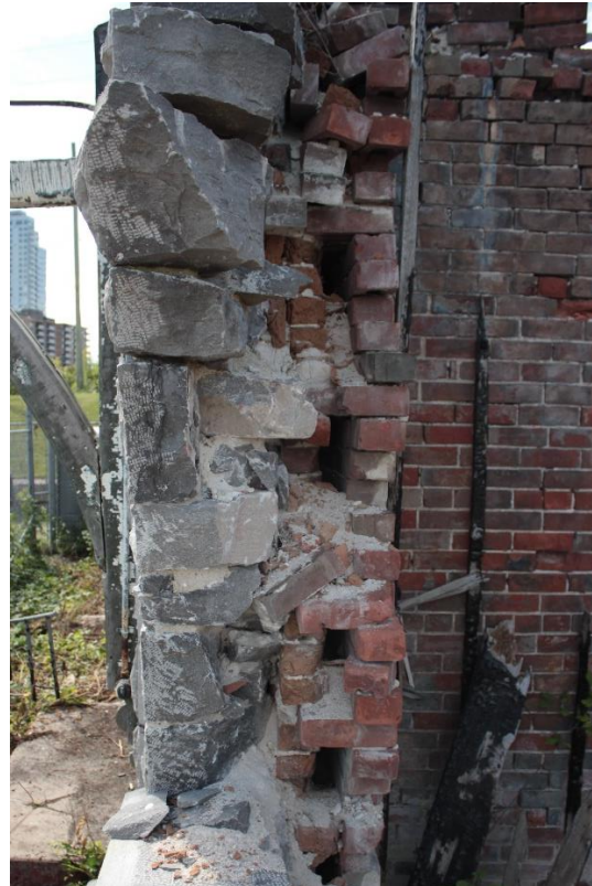
Figure 6: East wing wall assembly [JCAL 2021]
