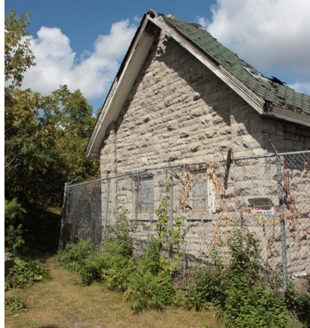
Figure 19: West wall exterior [JCAL 2021]
