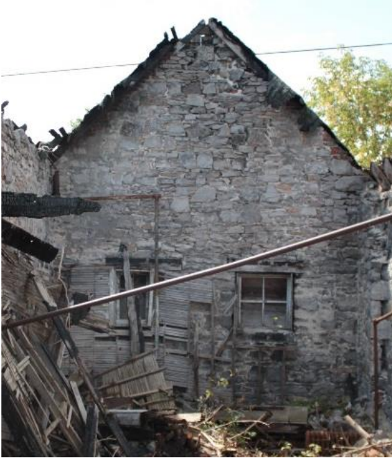
Figure 18: West wall interior [JCAL 2021]
