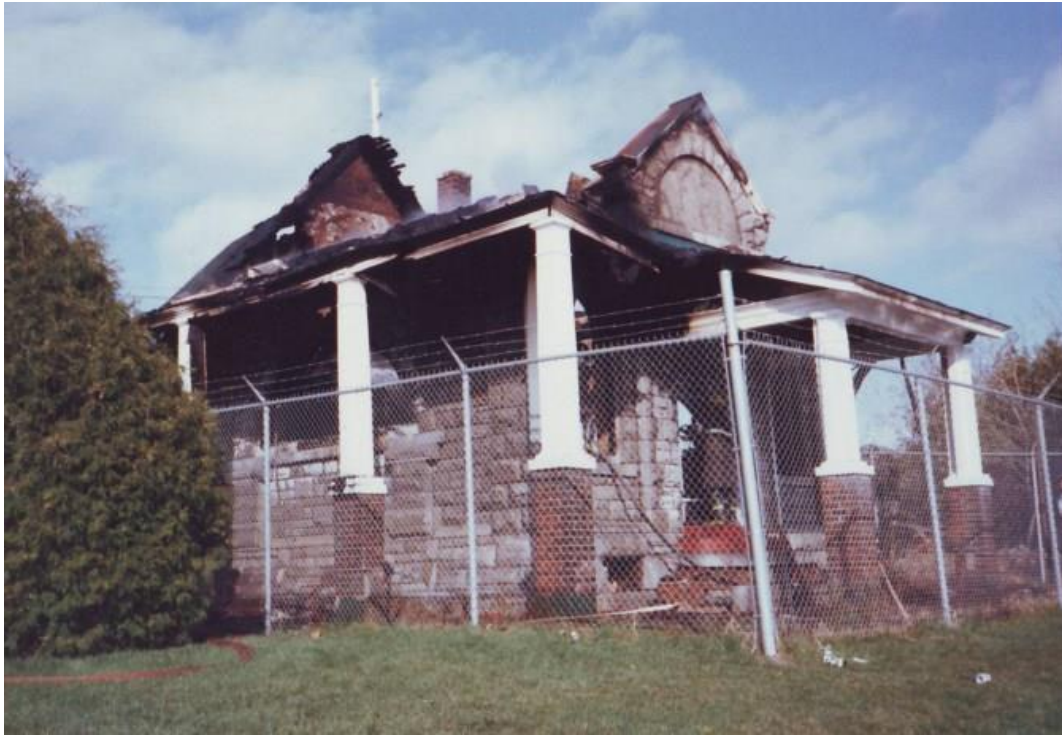
Figure 2: Hintonburg pumping station after 1989 fire
