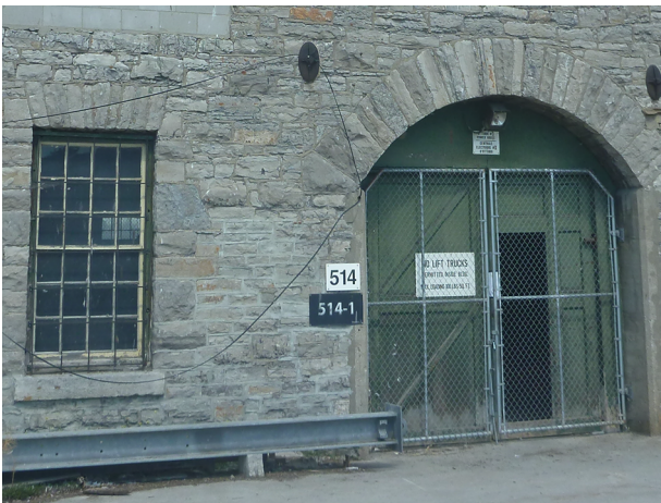
Figure 21: Original window and door (green) at Chaudiere Falls [JCAL 2015]
