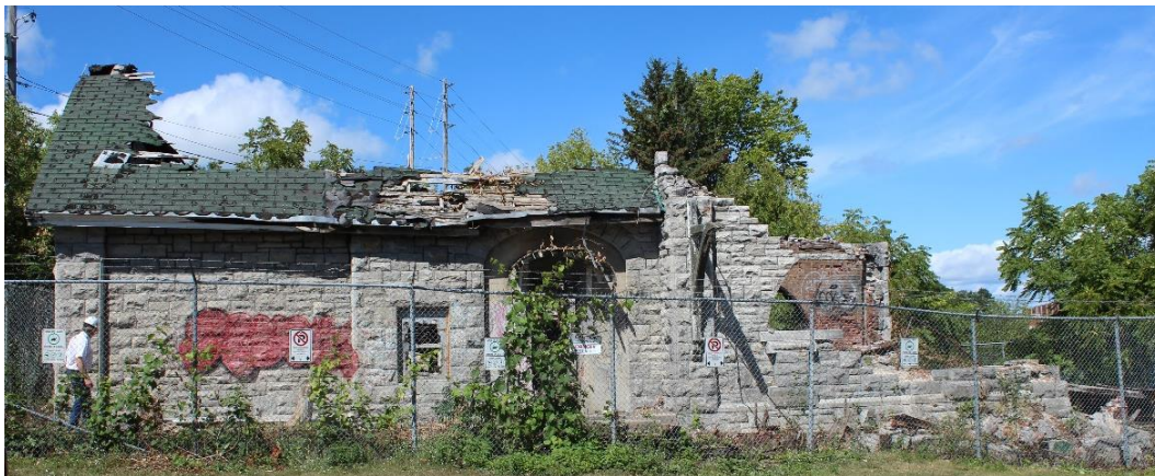
Figure 3: Hintonburg pumping station present day [JCAL 2021]
