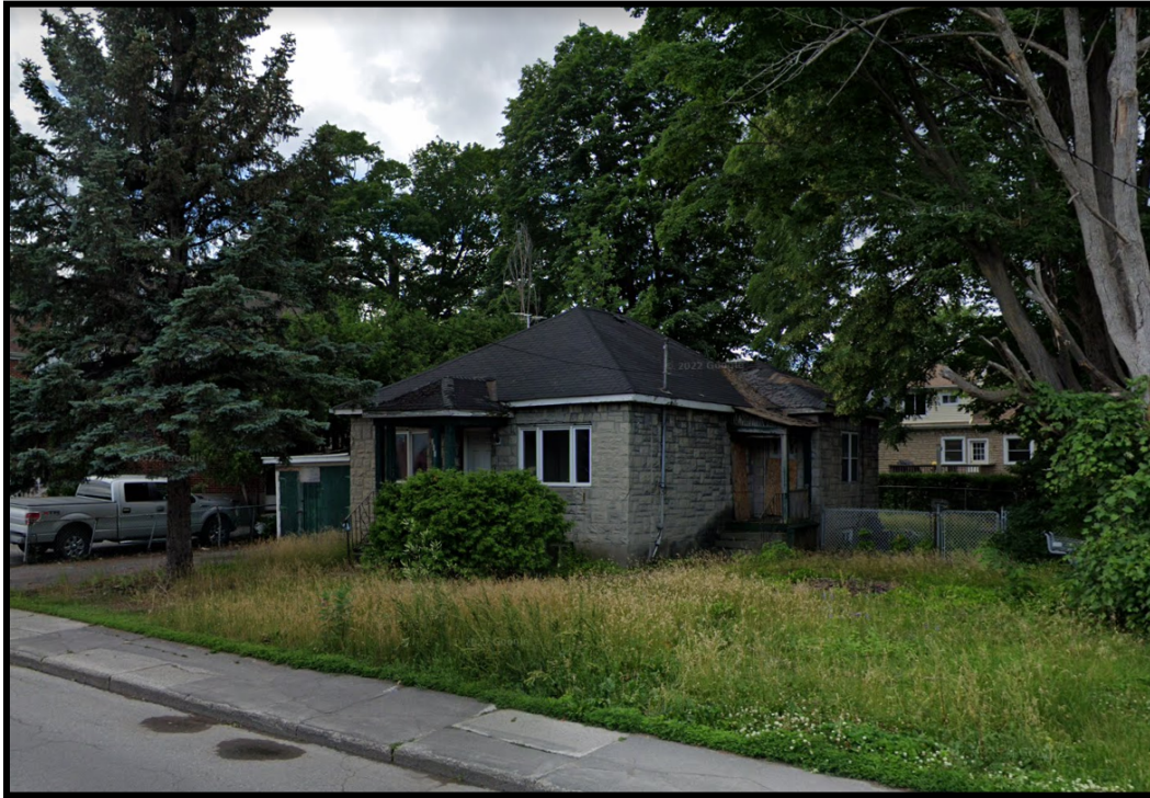
236 Woodroffe Ave. from Woodroffe Ave. looking south.
