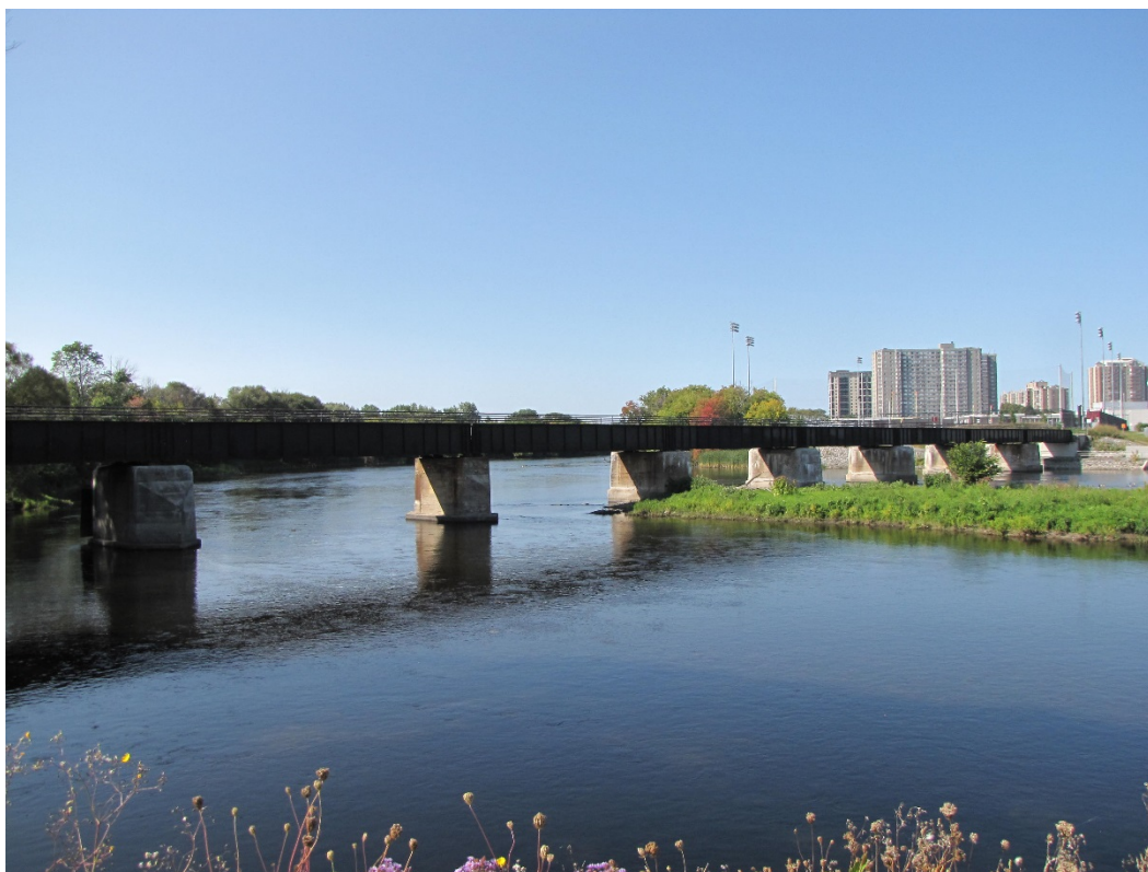
Photo 1 – North elevation of the Old Railway Rideau River Pedestrian Bridge. Note low-lying island downstream of Pier 5 and University of Ottawa (Lees Campus) located on west side of the river (background).
