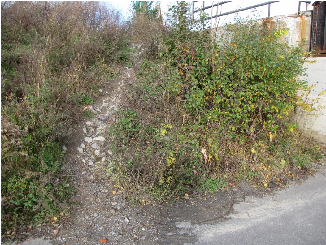
Photo 73 – Southwest embankment is well vegetated with light erosion due to a foot path leading down from the top of the embankment to the multi-use pathway below.
