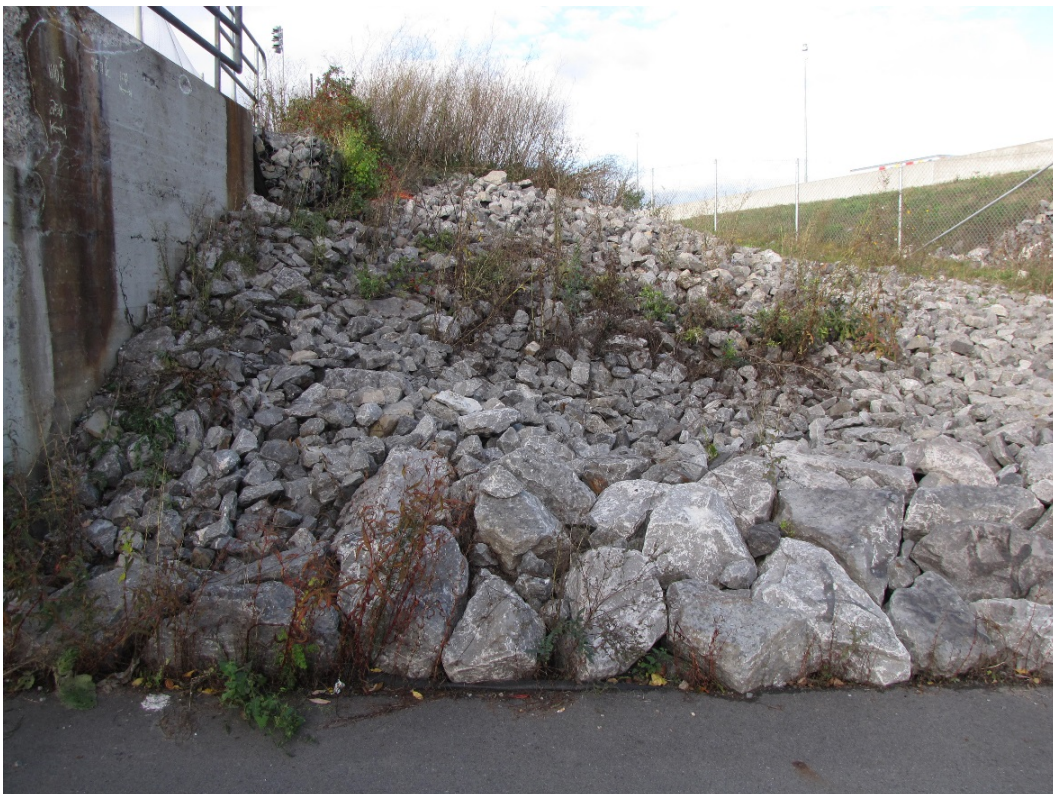
Photo 74 – Northwest embankment and rip-rap slope protection is in good condition.
