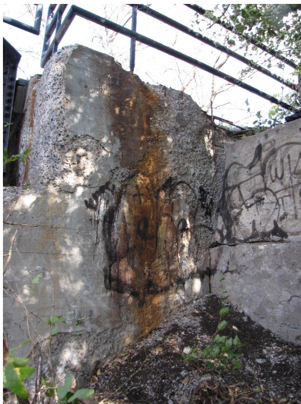
Photo 58 – Extensive areas of medium to very severe disintegration with exposed corroded rebar, delaminations, and hairline to narrow wet and efflorescence stained map cracking on the southeast wingwall.
