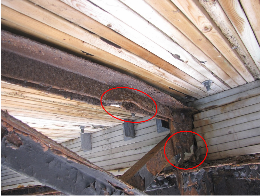
Photo 35 – Cross-frame 2 bays west of Pier 5. Perforation full width of the vertical gusset plate and severe deformation of the top brace member.
