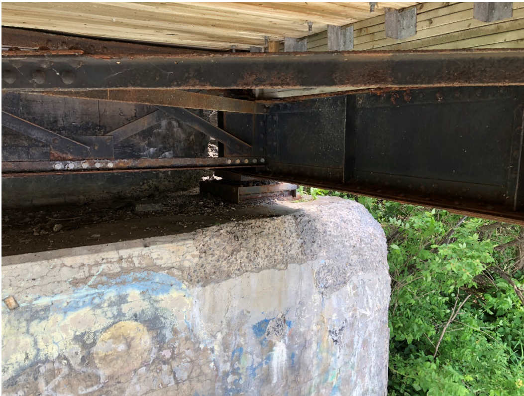
Photo 50 – Very severe disintegration at the top of the east abutment wall and bearing seat at the south end.
