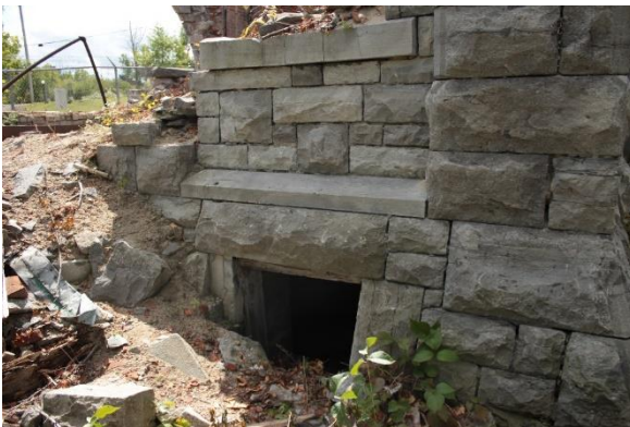
Figure 14: North basement on east wall [JCAL 2021]
