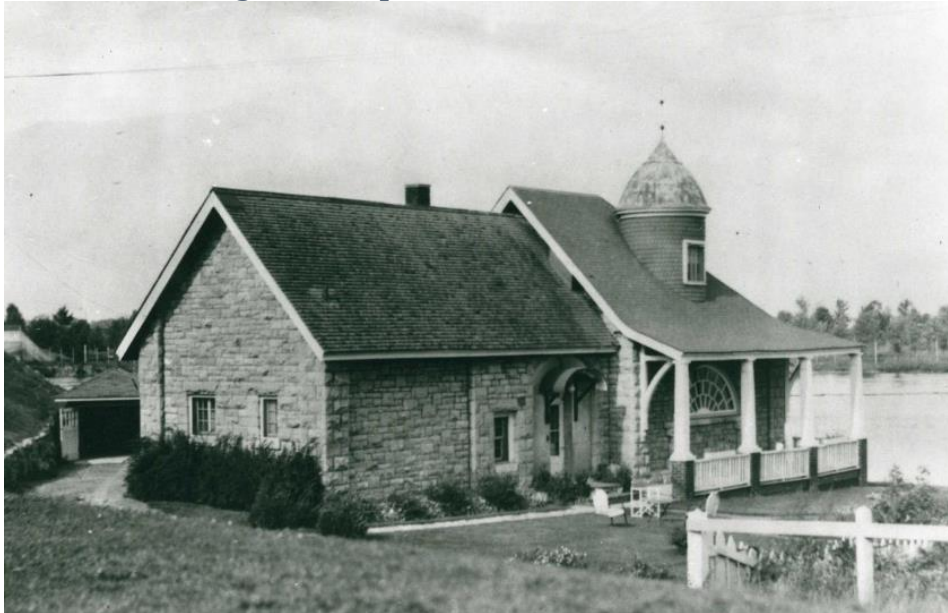
Figure 1: Hintonburg pumping station, 1928
