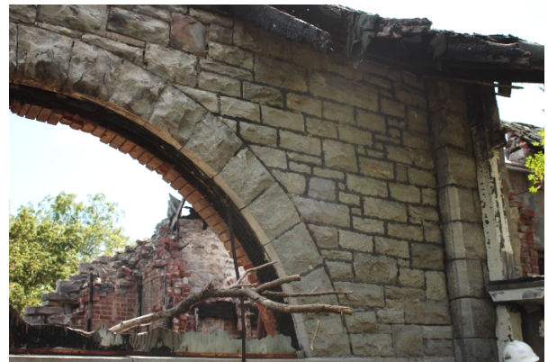
Figure 10: Repointed limestone masonry around arch [JCAL 2021]
