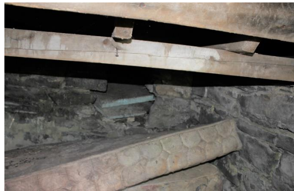
Figure 15: Basement interior [JCAL 2021]
