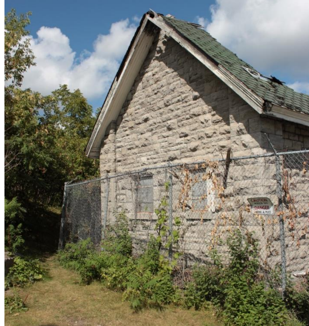
Figure 19: West wall exterior [JCAL 2021]
