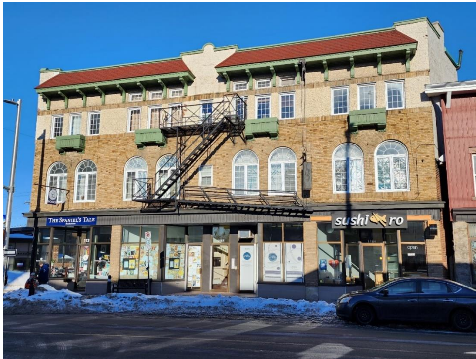
Front Façade Source: City of Ottawa, 2023
