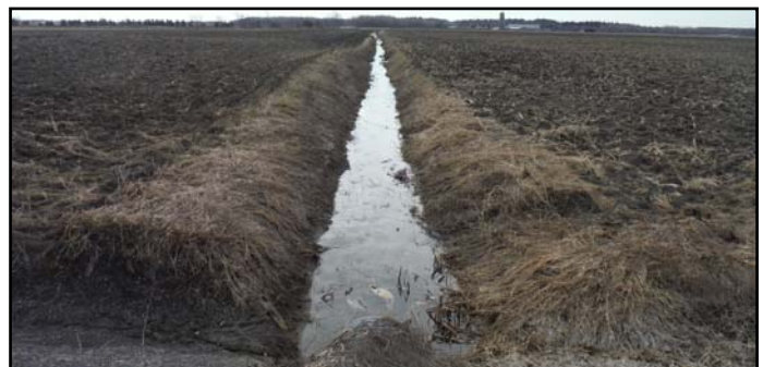
Channelized drainage feature on Regimbald Road
