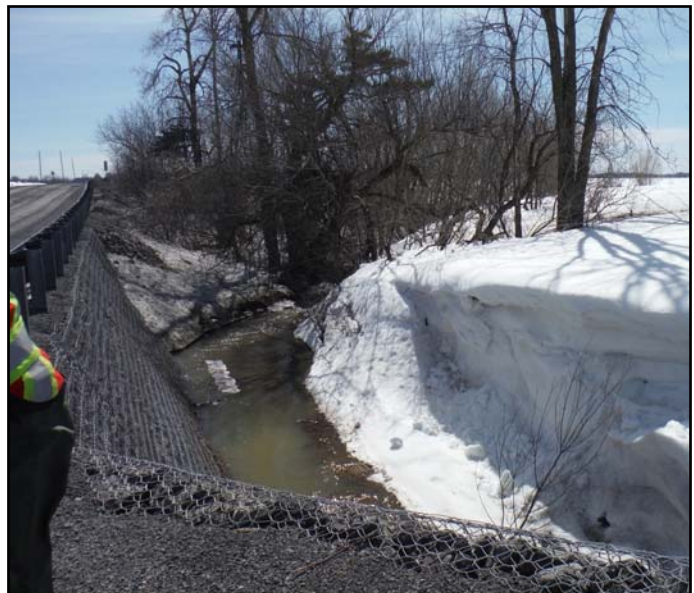
An example of mixed modifications: channel straightening and hardening with gabion baskets on Birchgrove Road
