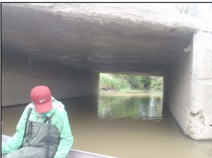
Road crossing altering riparian zones along Becketts Creek
