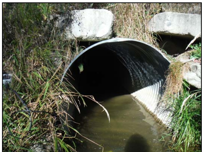
A highly altered stream section flowing through a culvert
