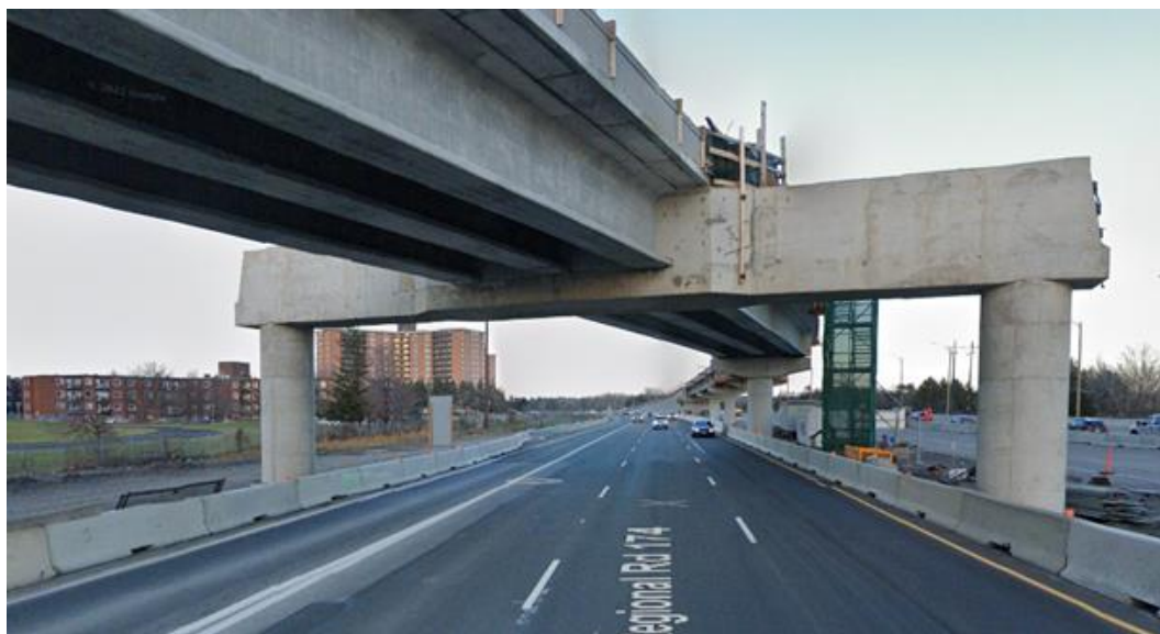
Figure 2B – Example of Straddle Bent Structure
