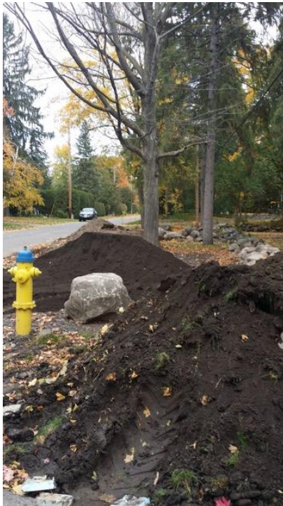
Figure 3-A: City of Ottawa while using the front yard to store landscaping materials during sewer constructions removed sections of the loose stone wall. Note buried wall and soil piled up on tree roots.
