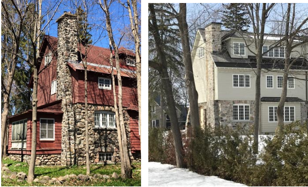
Figure 4-A: Comparison of the building before and after. G. Statler Construction Record.
