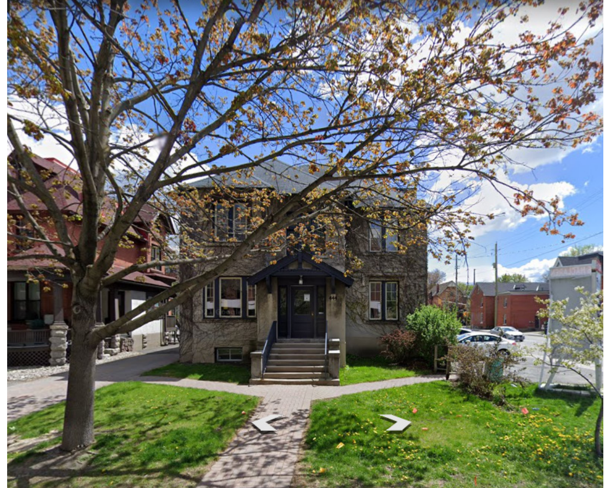
Current Heritage Home, 444 MacLaren Street
