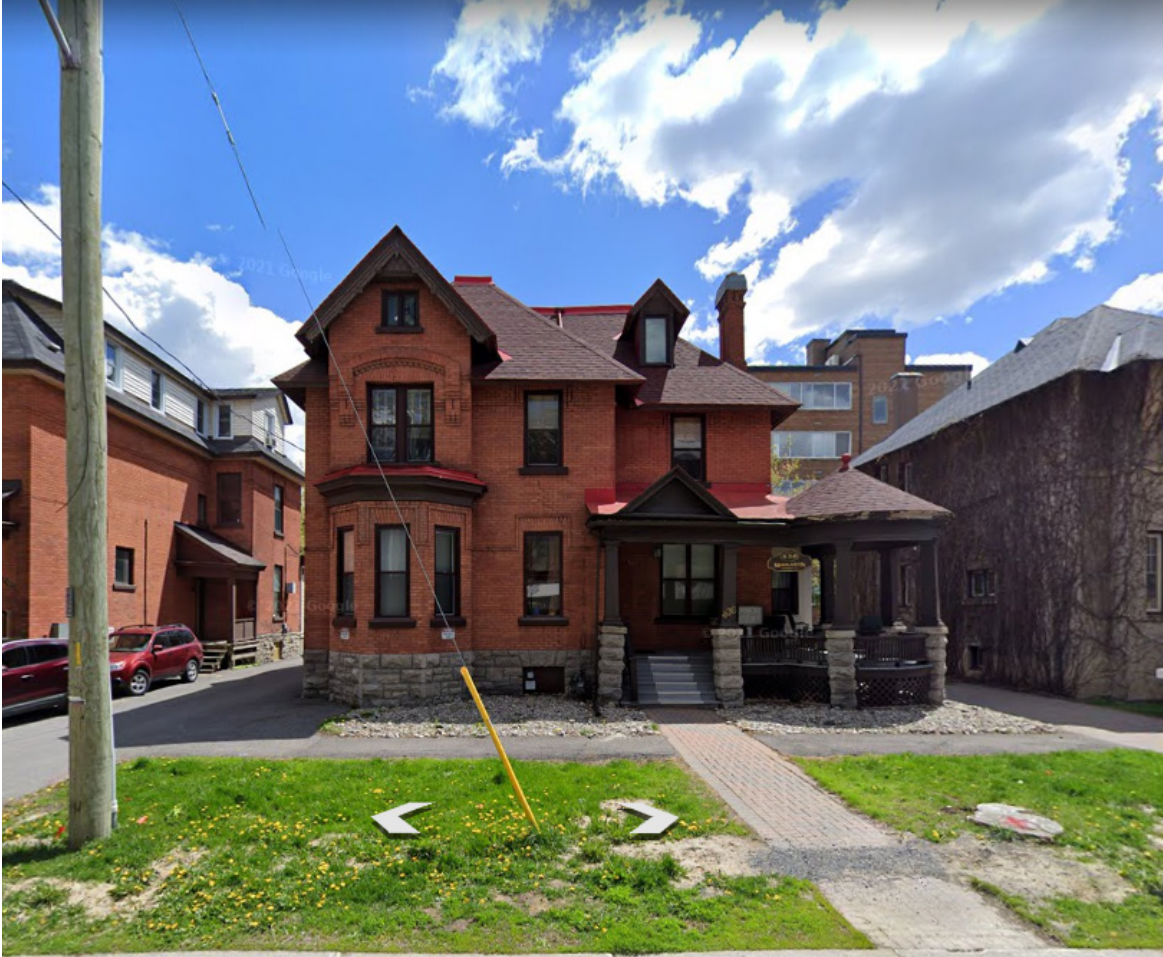
Current Heritage Home, 436 MacLaren Street
