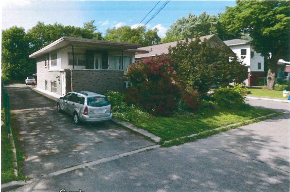
365 St Denis Street (foundation encloses entry to lower unit, 2.19 m from lot line)
