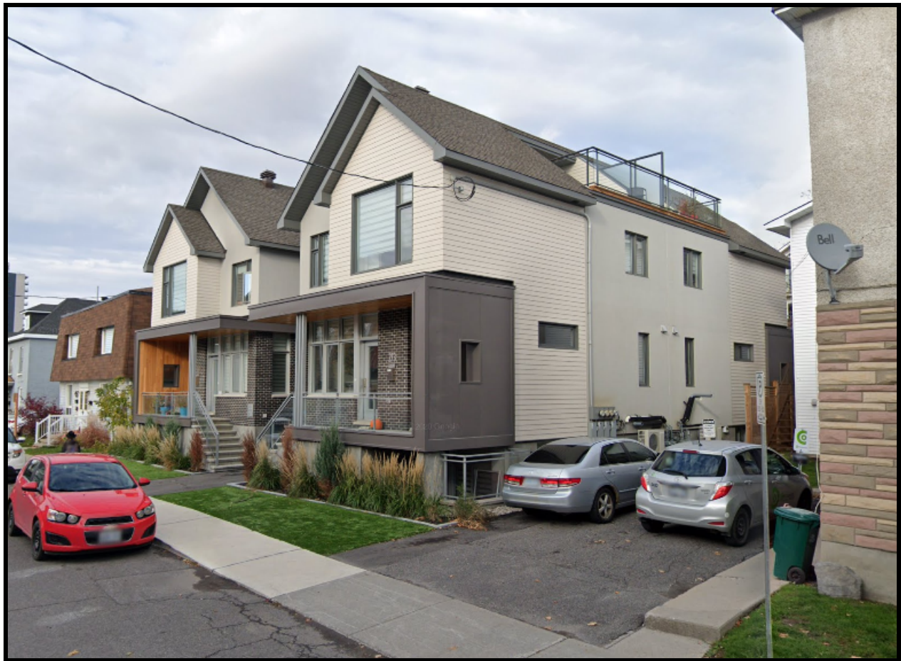
Figure 4. 267, 269, 271, and 273 Carruthers, two sets of semi-detached dwellings with SDUs built between 2017 and 2019. Each primary dwelling has a parking space located in the rear yard accessed via a central single lane driveway. Note the vehicle forced to park in the street, and the vehicles parked to the right of the houses.
