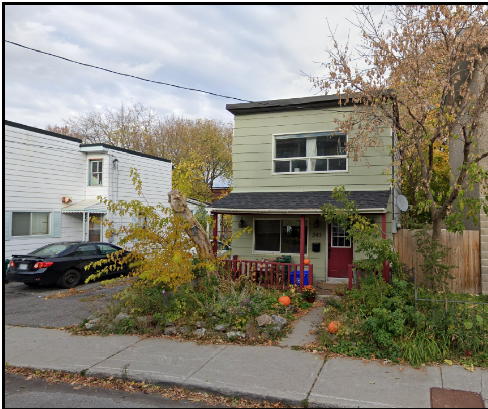
Figure 1. 243 Carruthers, a 2-story single detached dwelling, looking north.
