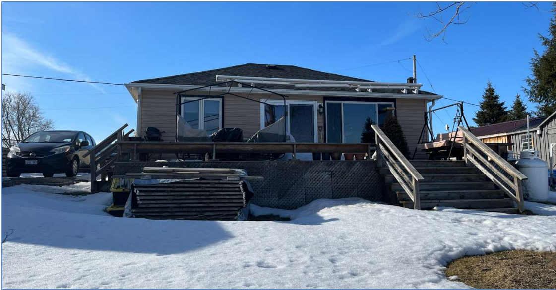
Exhibit E-2: Photograph of the rear of the Subject Property (March 24, 2023)
