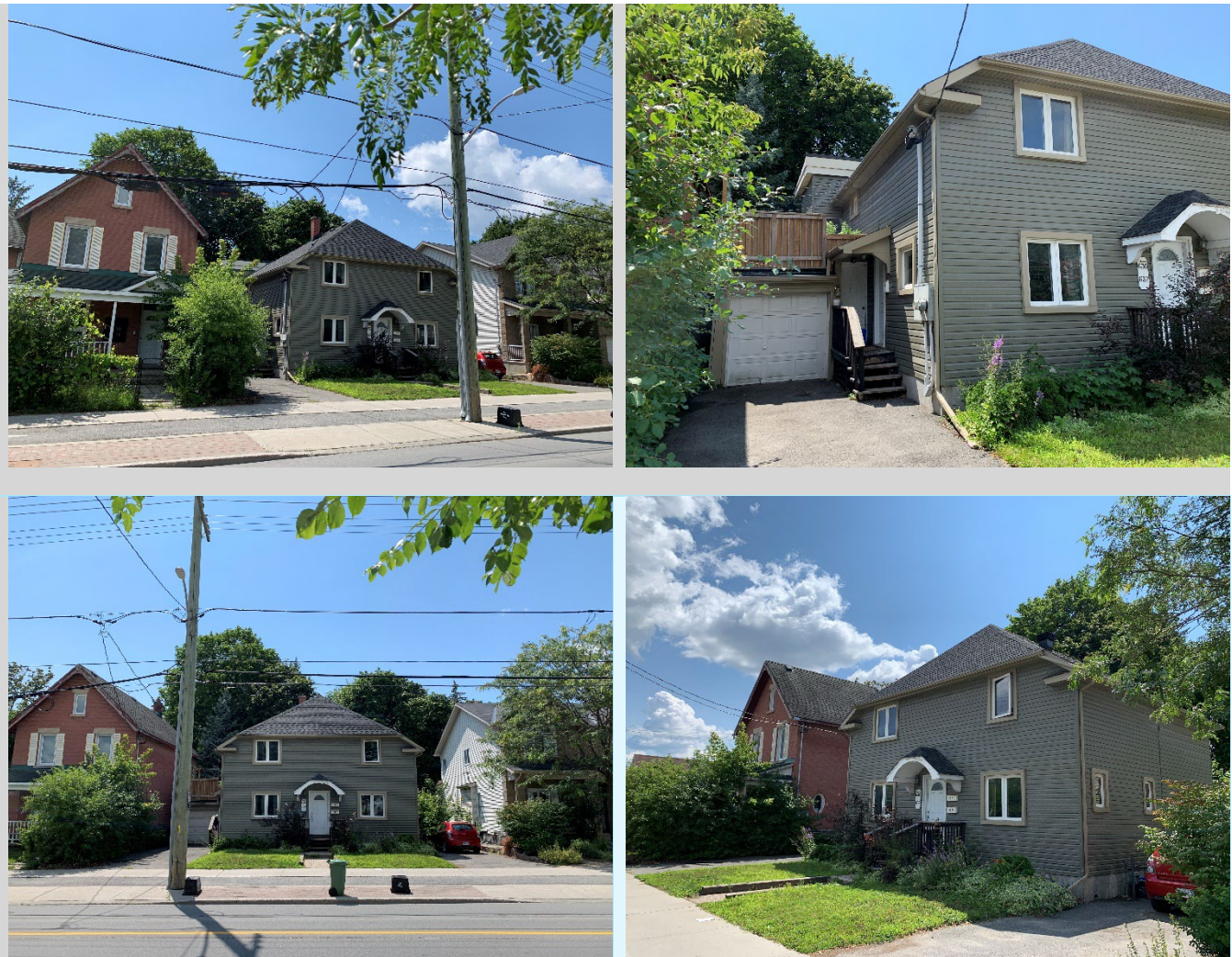
Figure 1: Top Left, looking northwest towards the subject property; Top Right, looking west towards the southern portion of the subject property; Bottom Left, looking west directly towards the subject property from across Churchill Avenue North; Bottom Right, looking southwest towards the subject property.
