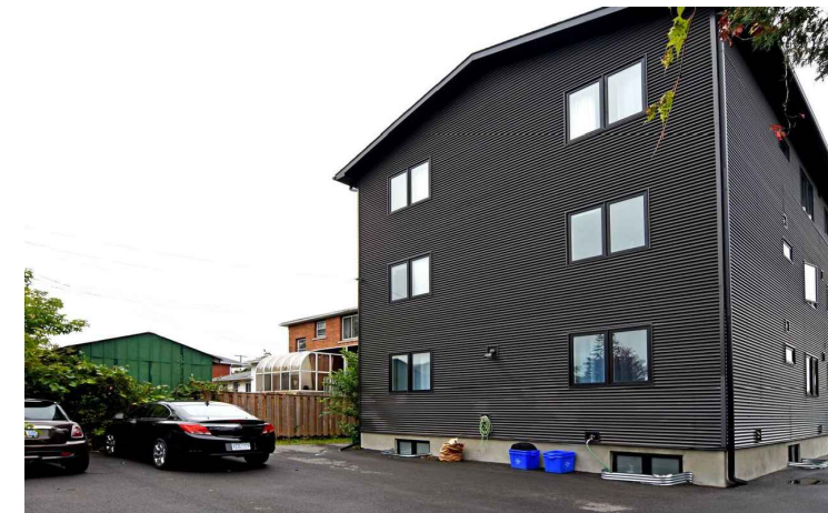
3 STOREY APARTMENT 279 GLYNN
