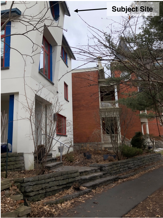
Image 2. Subject site looking northwest from NCC multi-use pathway along Queen Elizabeth Driveway (2023)
