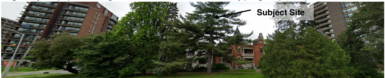
Image 7. Subject site and adjacent properties looking west from Queen Elizabeth Driveway (Google Maps, 2022)
