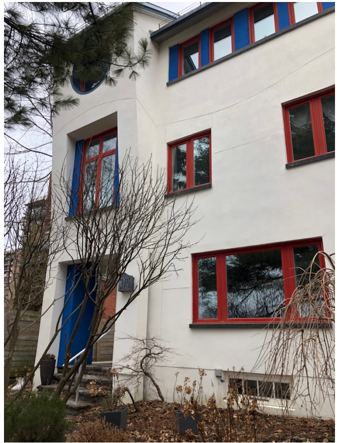
Image 3. Subject site looking north from NCC multi-use pathway along Queen Elizabeth Driveway (2023)
