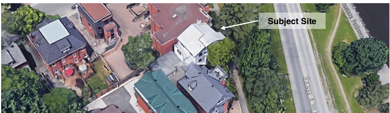
Image 8. Aerial imagery of subject site looking north (Google Maps, 2022)
