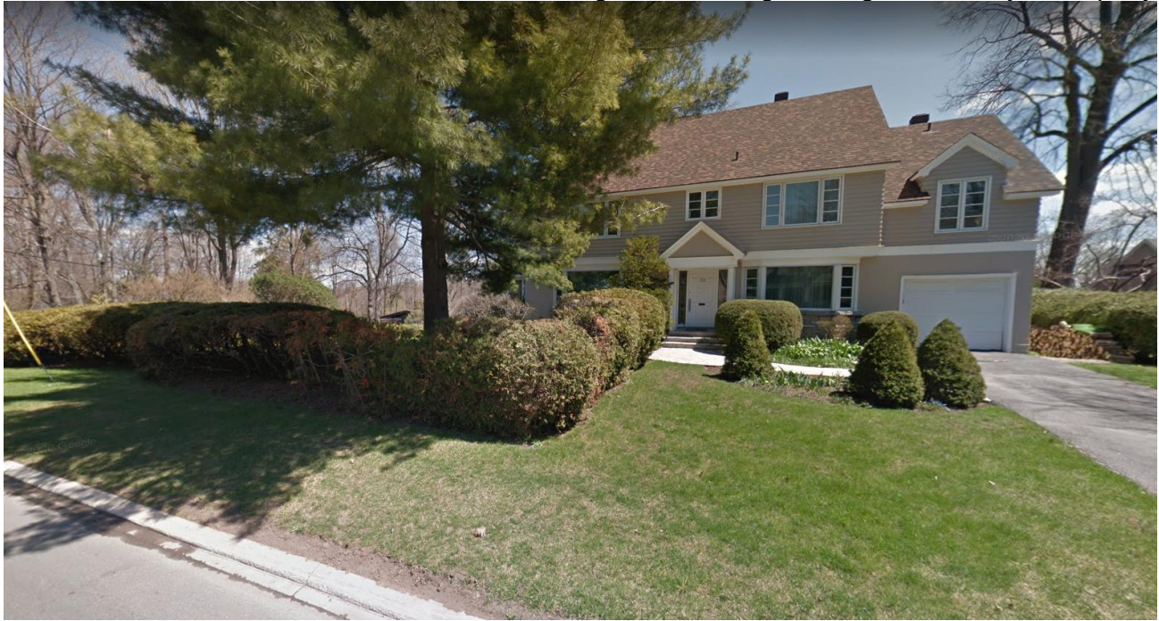
Figure 3: Existing Building on the Subject Property
