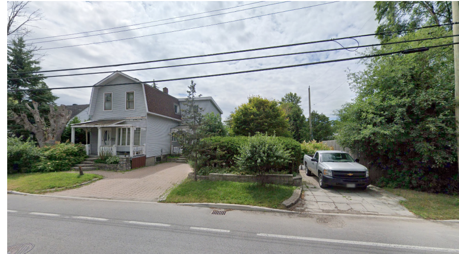
STREET VIEW OF SITE FROM KILBORN AVENUE
