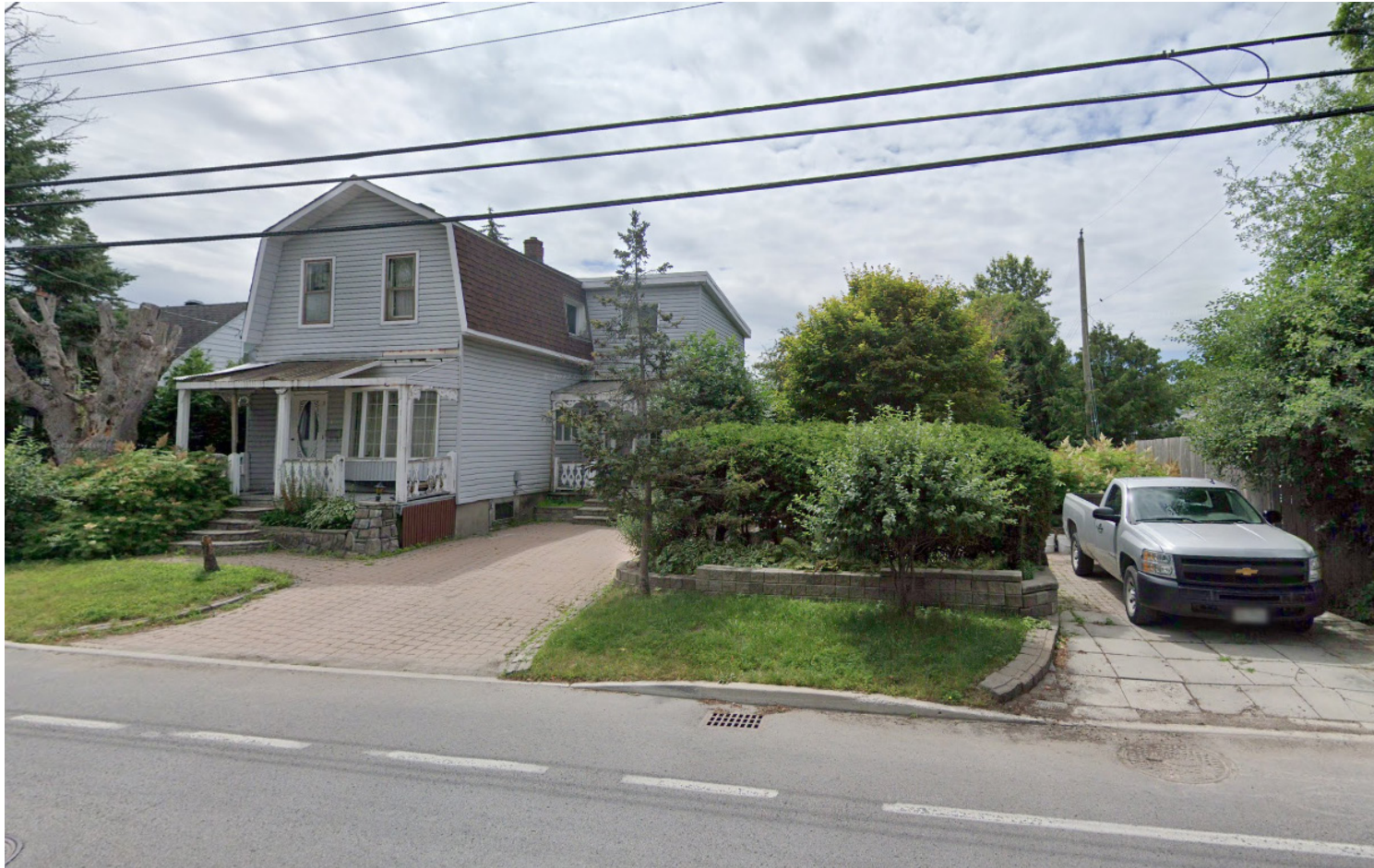
STREET VIEW FROM KILBORN AVENUE - EXISTING
