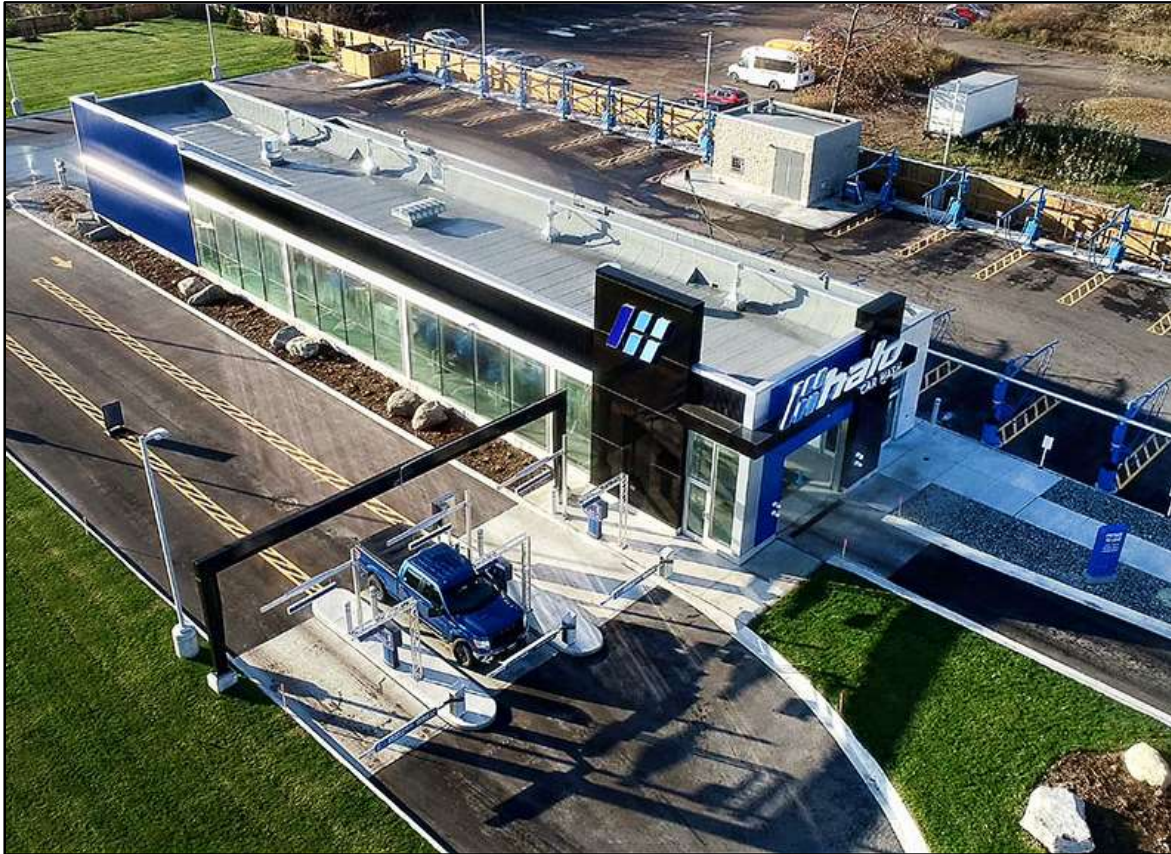
Exhibit J: Typical Halo Car Wash layout with three queuing lanes and entrance arch (foreground), wash tunnel and vacuum stalls (background) (Pictured: 3604 Innes Road, Ottawa)
