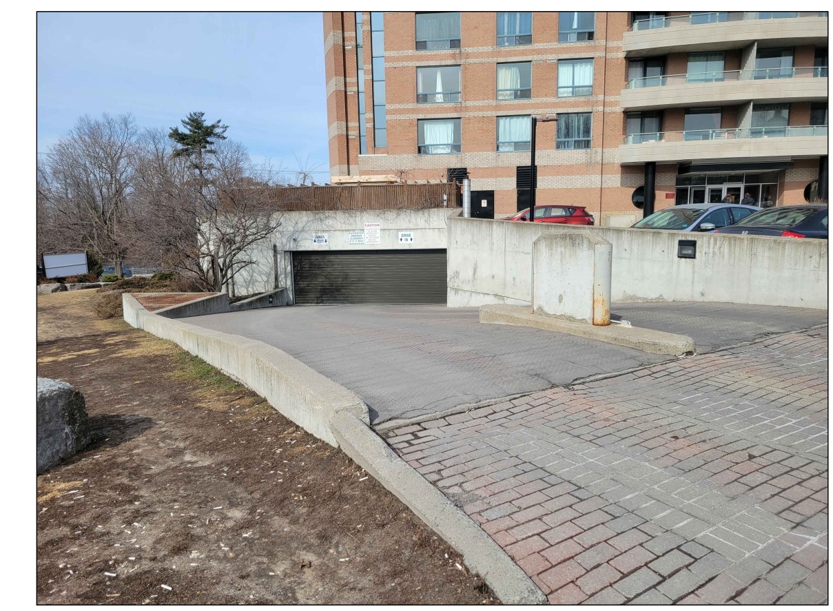
CURRENT VIEW OF RAMP LOOKING WEST
