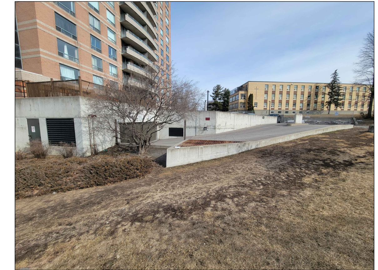
CURRENT VIEW OF RAMP LOOKING NORTH
