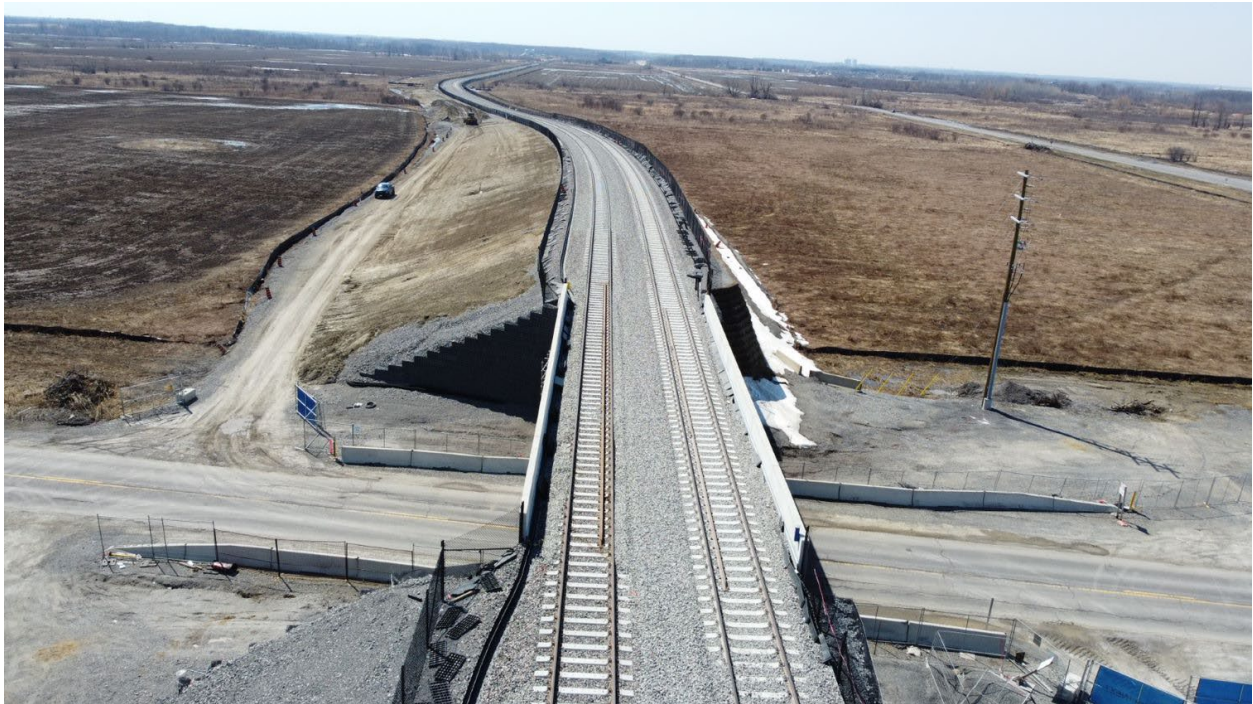
Figure 4: Ballasted Track at Bowesville Road
