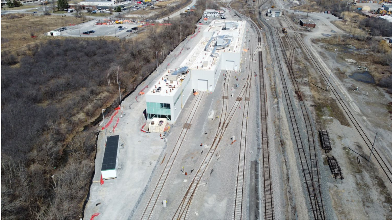
Figure 7: Albion Yard Maintenance and Storage Facility
