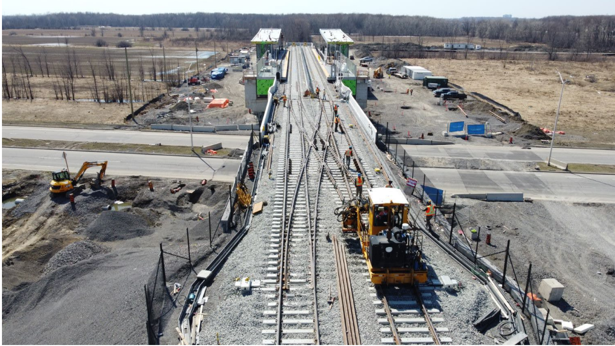
Figure 6: Elevated Diamond Crossover at Limebank Station
