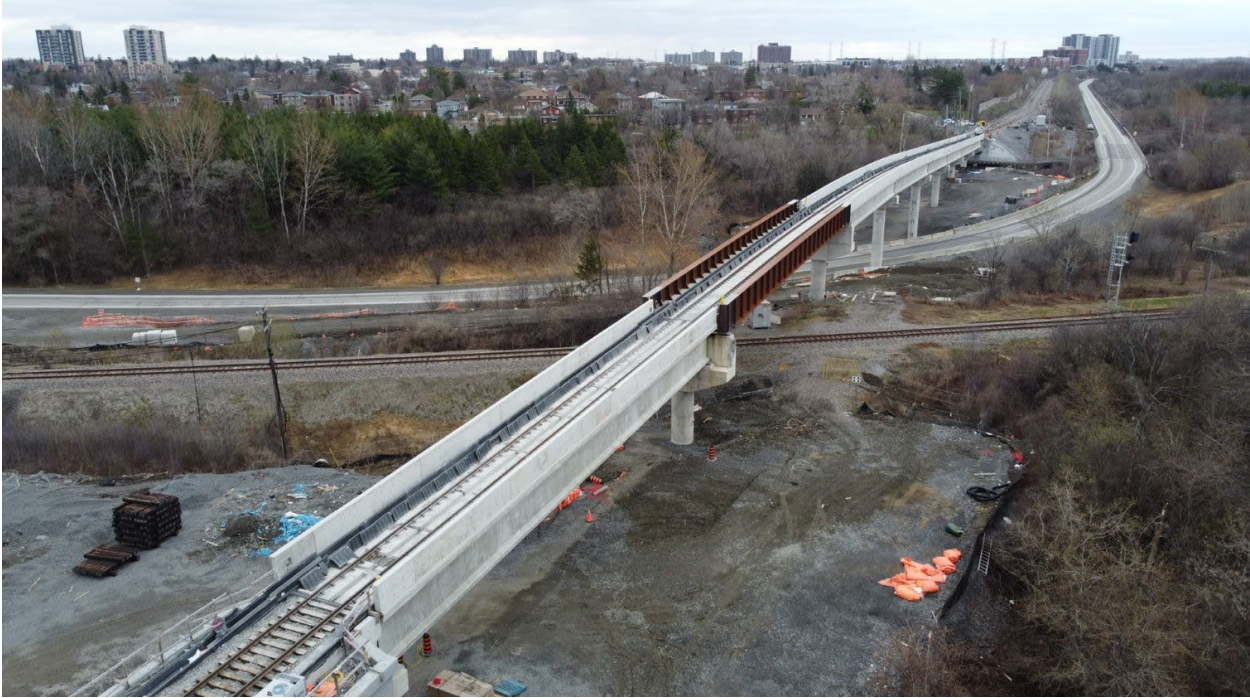
Figure 5: Direct Fixation – Ellwood Grade Separation
