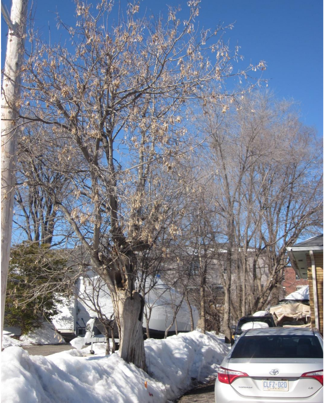
Picture 1. Tree #1, hazardous Manitoba maple at 259 Glynn Avenue
