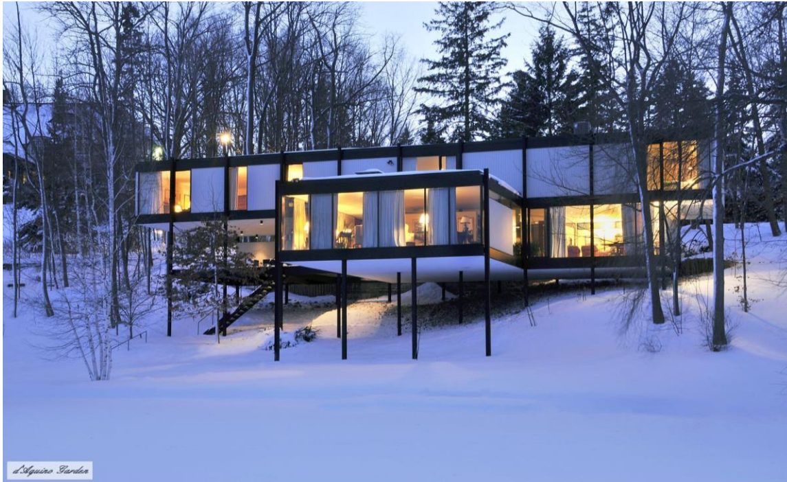
Figure 7: Winter view of the Hart Massey House is an art piece in the landscape overlooking MacKay Lake. This distinct residence just one block east of the subject property illustrates the eclectic range of styles that Rockcliffe Park features. Attributes of the residence such as the raised floor on stilts, clean lines and modularity are suggested in the proposed Cloverdale project. Source: Thomas d'Aquino. http://thomasdaquino.ca/house-and-garden/
