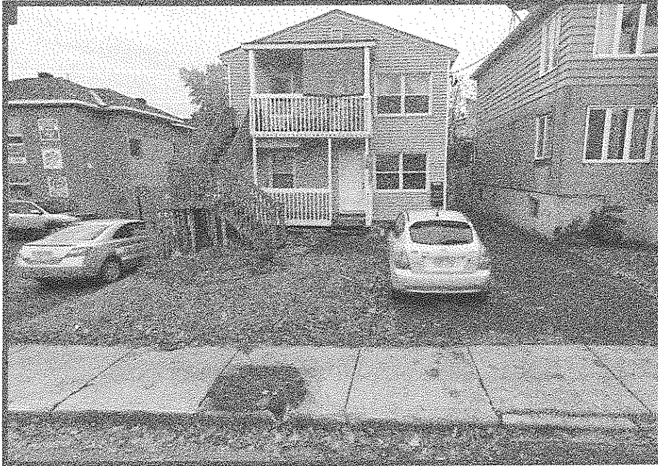
Front yard parking at 298 Montfort which is a triplex building.
