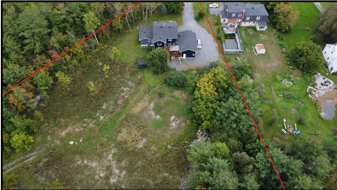
Aerial photo showing the interior of the lot and the existing detached dwelling fronting on Campbell Reid Crt with the approximate site outline . (Sept. 2022 photo).
