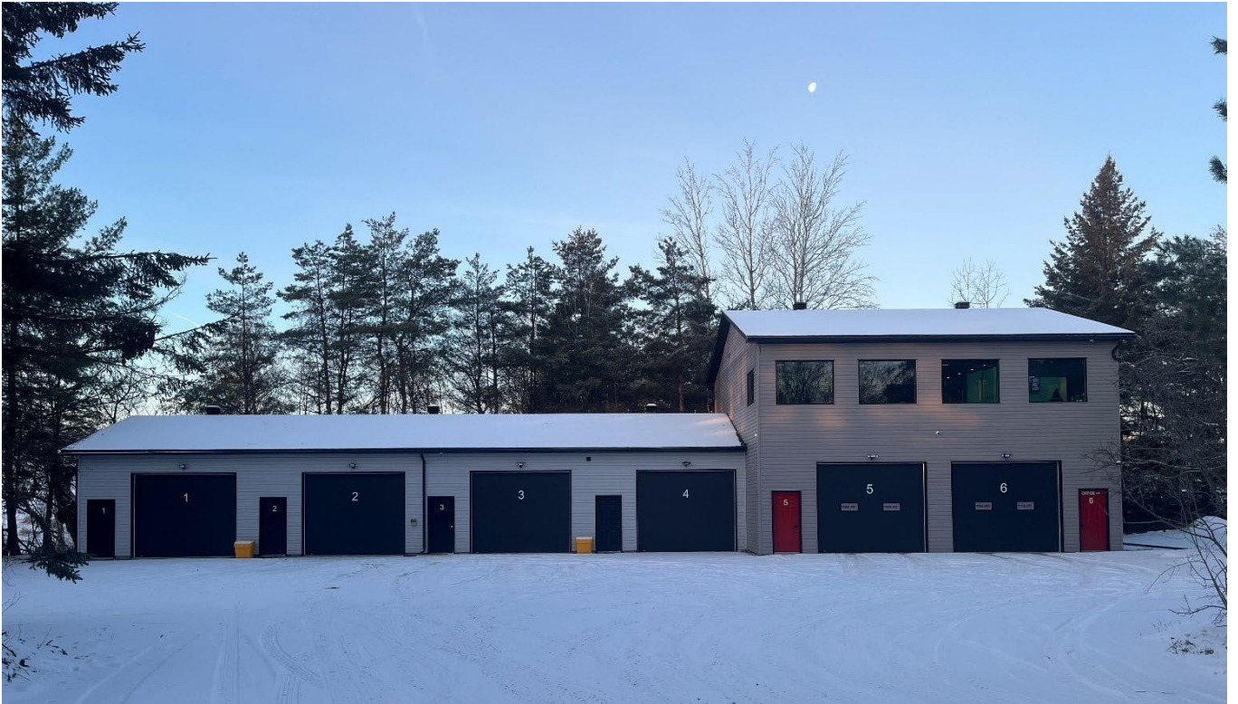
Image 2: Photograph of front façade of the existing warehouse and office building.
