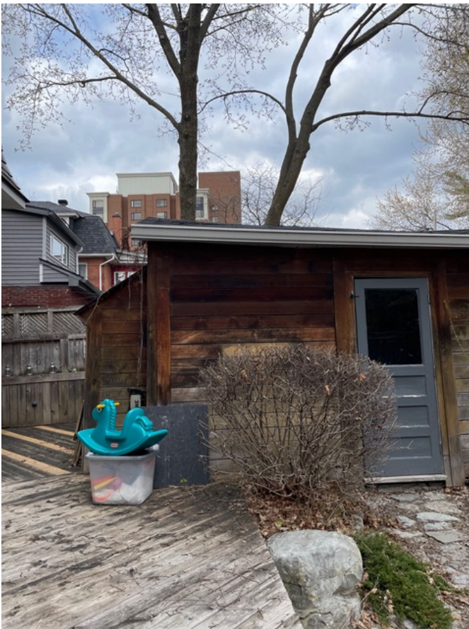
Image 5. Rear yard conditions looking east towards the side façade of existing garage
