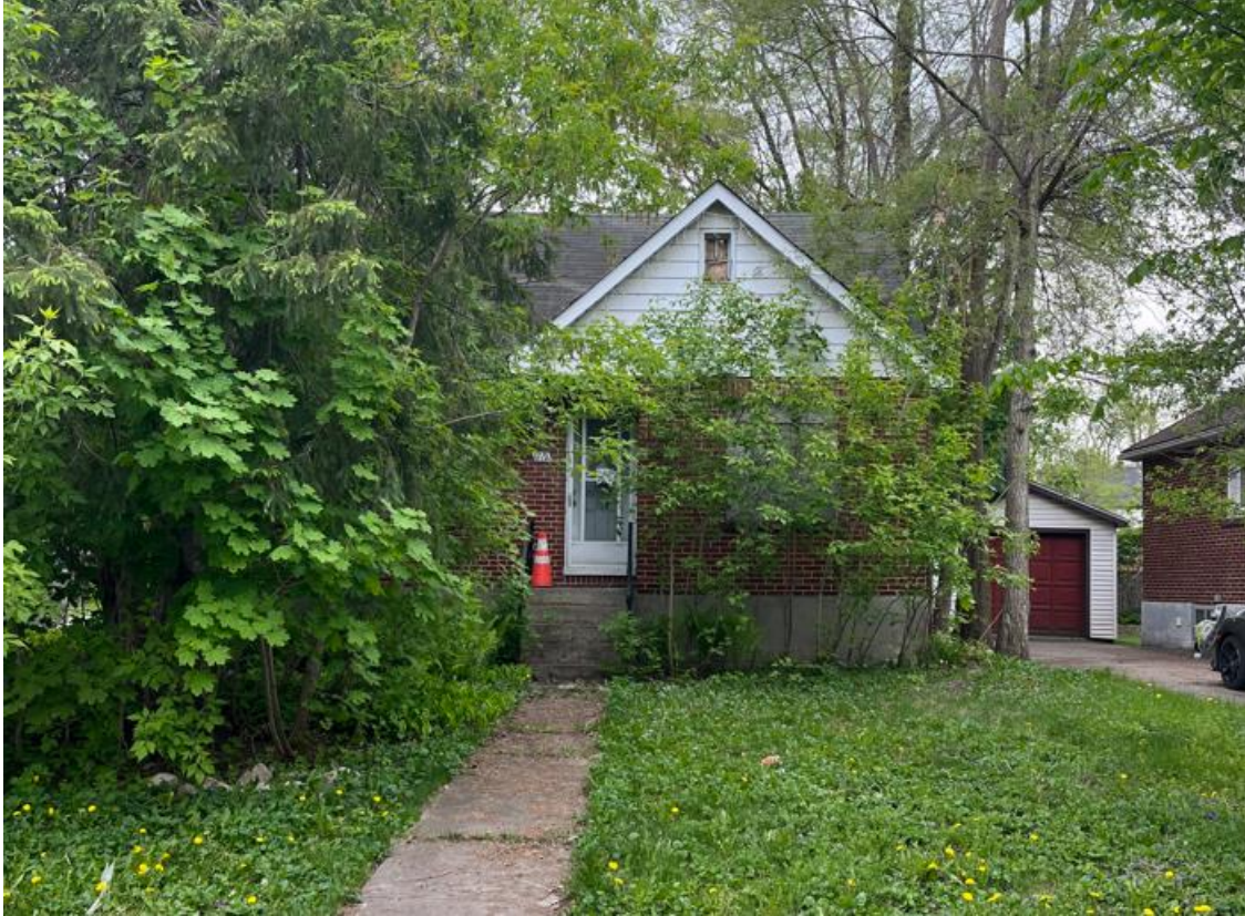
Figure 3: Existing Building on the Subject Property
