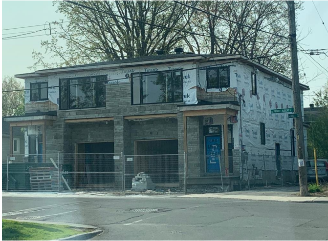
Figure 2. Current construction of semi-detached homes
