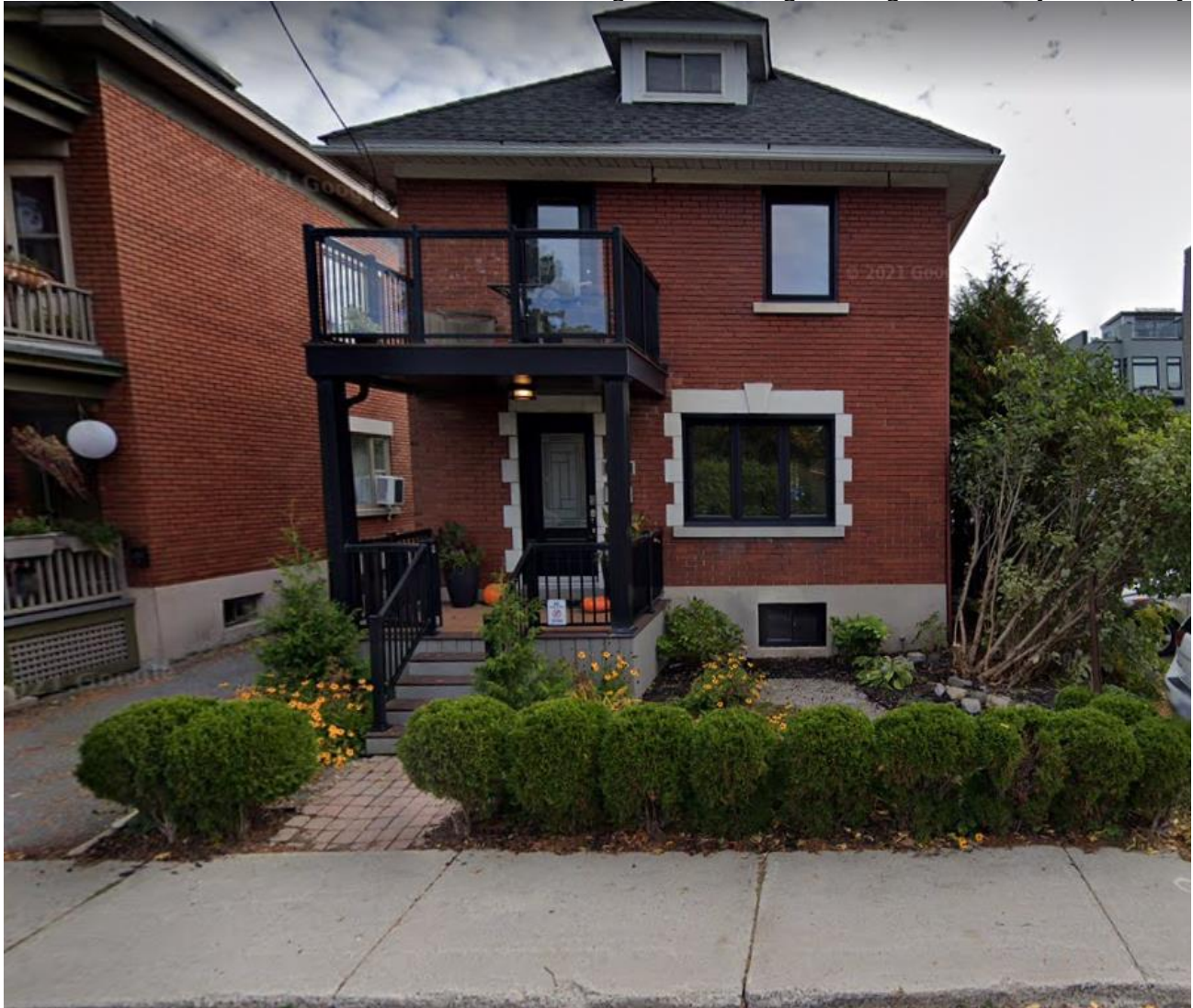
Figure 3: Existing Building on the Subject Property
