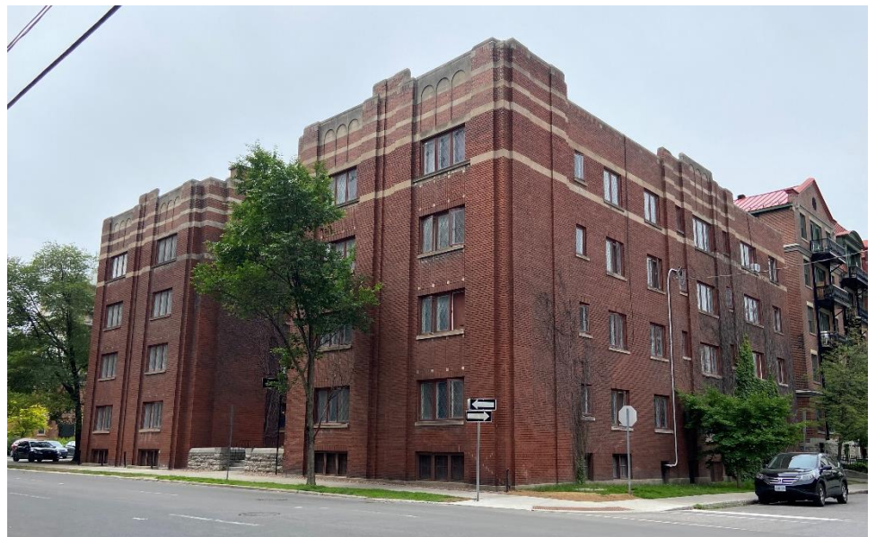
46 The Duncannon, designated under Part IV of the Ontario Heritage Act. MTBA
