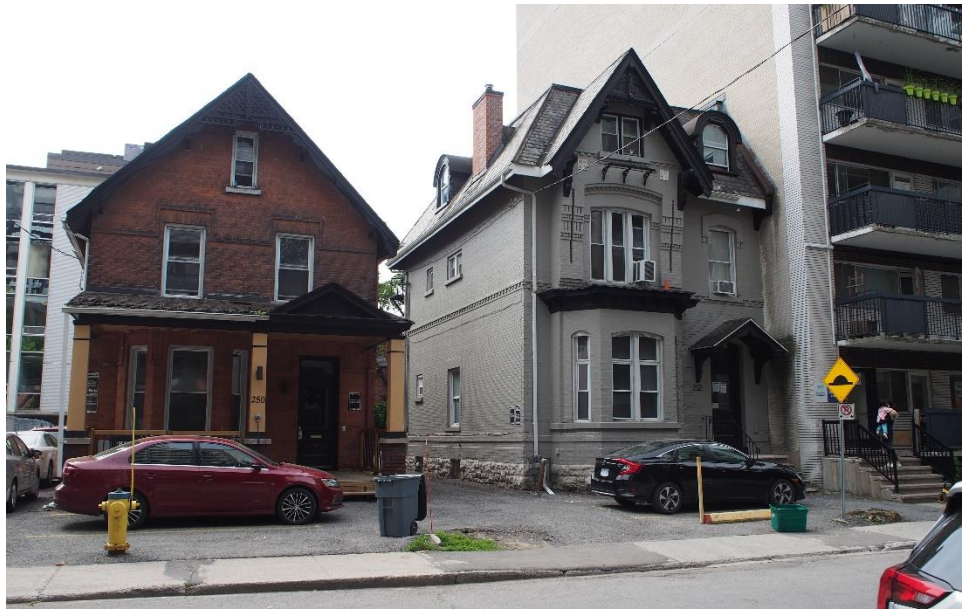
20 View of 250-252 Lisgar Street located west of 230-232 Lisgar. MTBA
