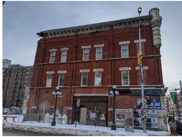
Figure A2 – North Exterior Wall
