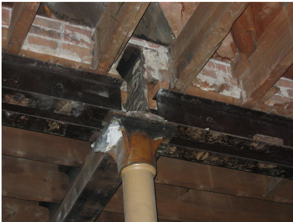
Figure 3: Previously Existing Condition Brick Partition Walls
