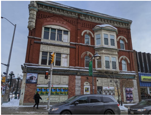
Figure A1 – West Exterior Wall
