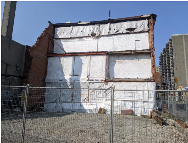
Figure A3 – East Side of the Building
