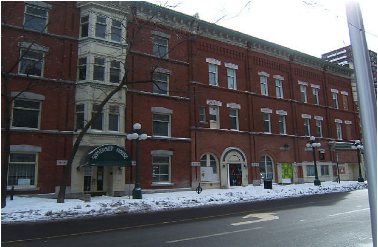
Figure 2: Previously Existing Condition Showing Eastern Addition
