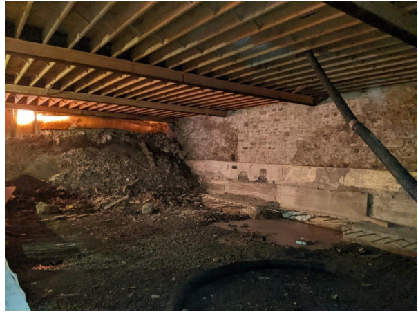
Figure A6 – Basement South Foundation
