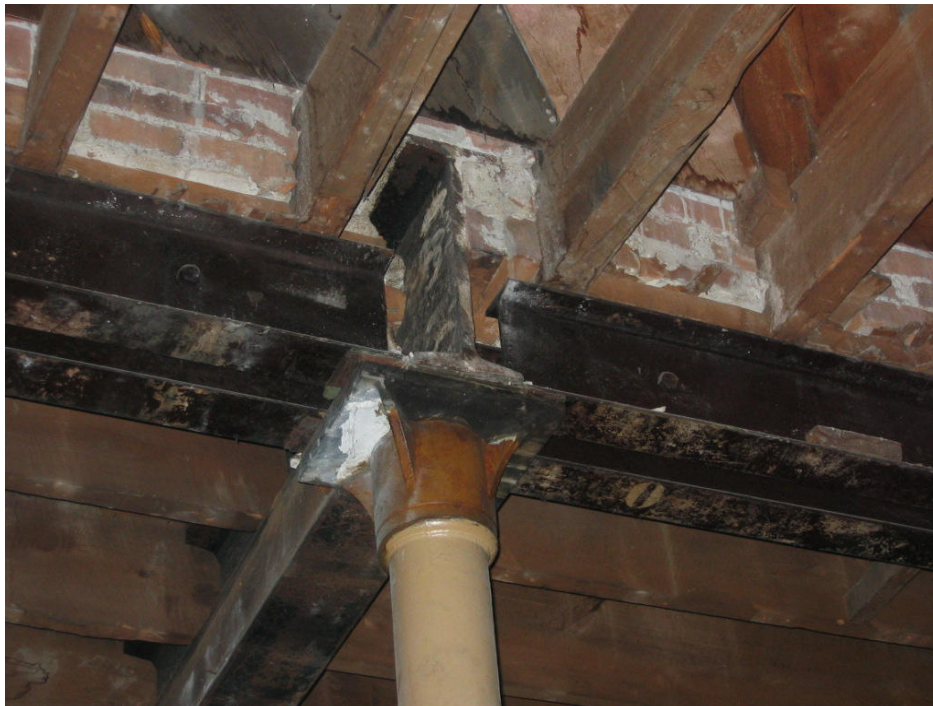
Figure 3: Previously Existing Condition Brick Partition Walls
