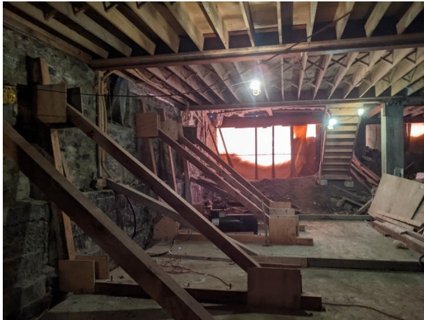
Figure A5 – Basement North Foundation
