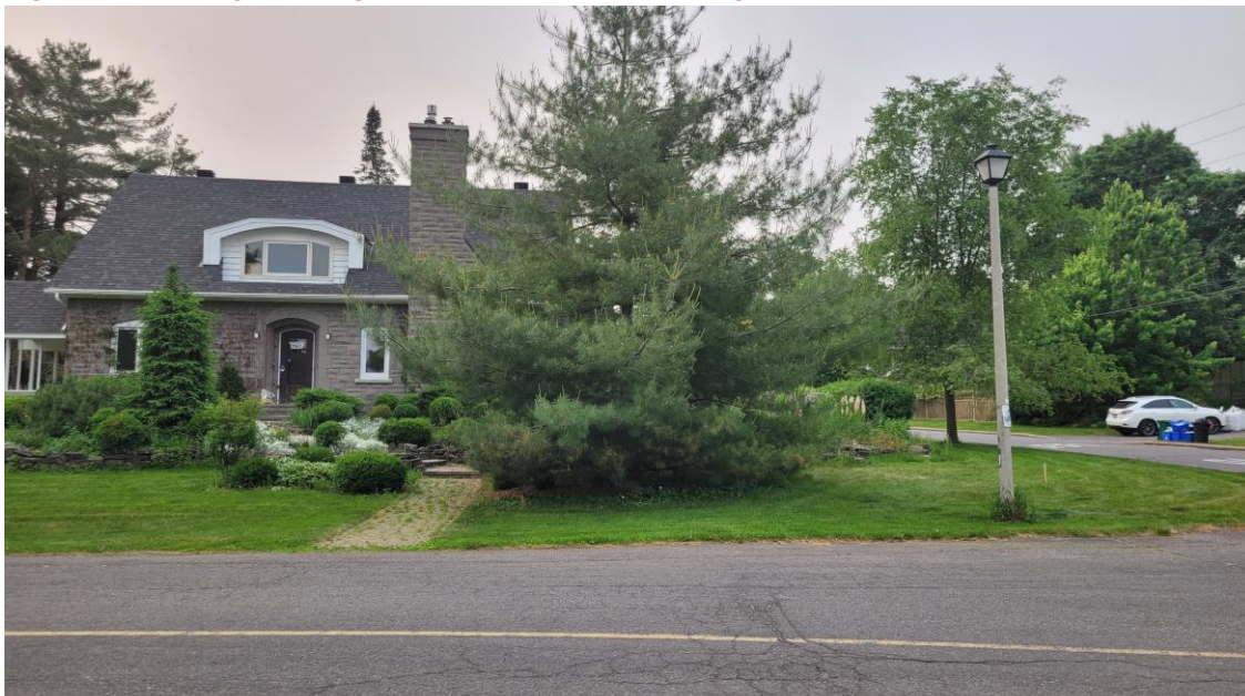
Figure 1-3: Existing dwelling at 1469 Portal Street, looking south
