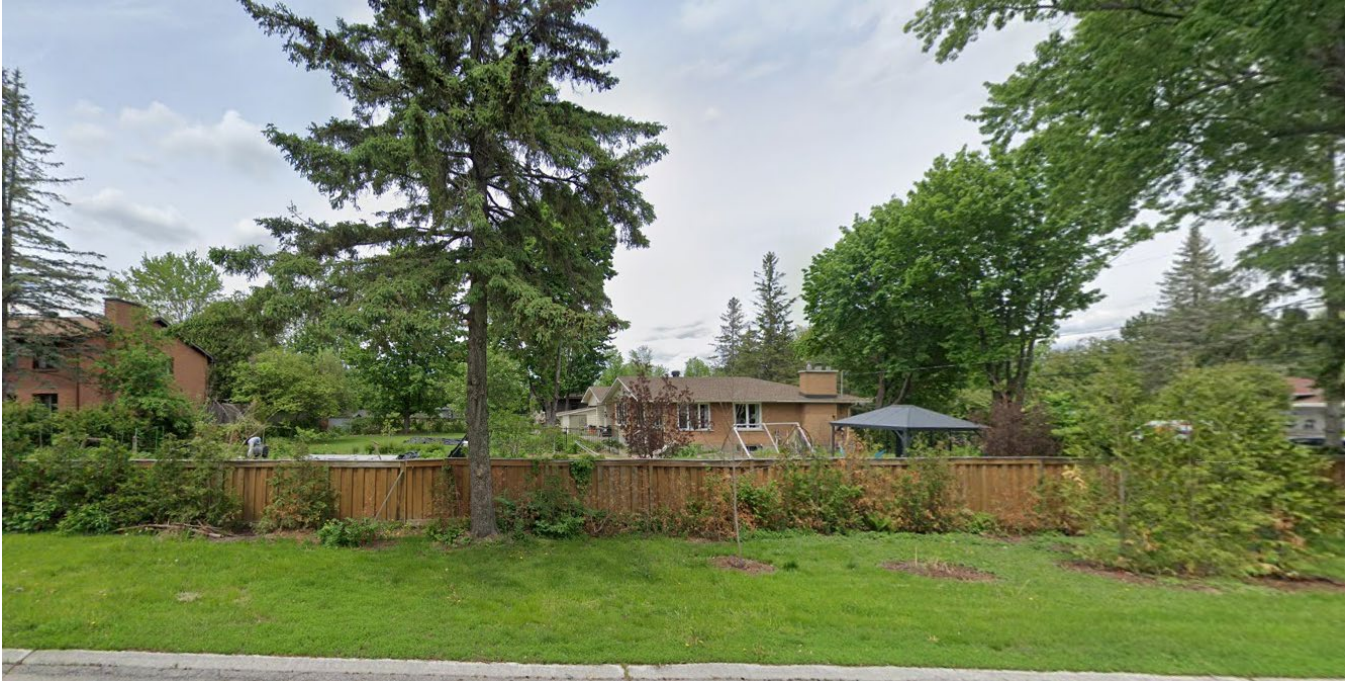
Figure 5. View of the subject property from Massey Lane
