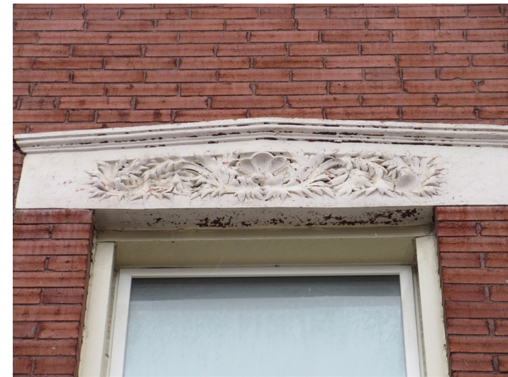
Precast Stone Window Headers to be Restored
