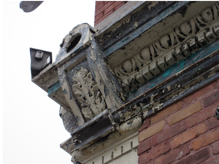
Cornice Brackets to be restored
