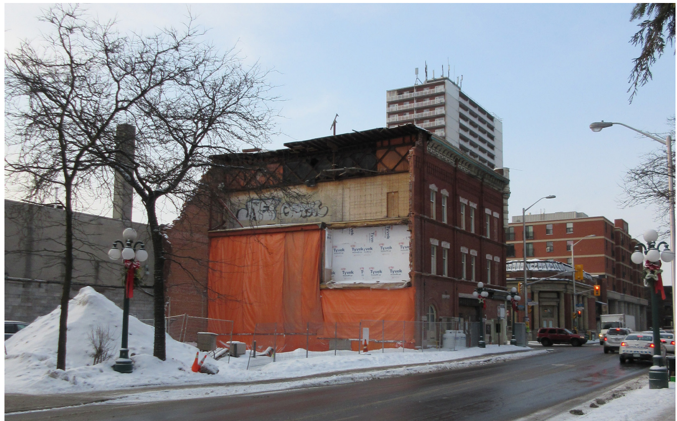
Existing structure at Somerset Street
