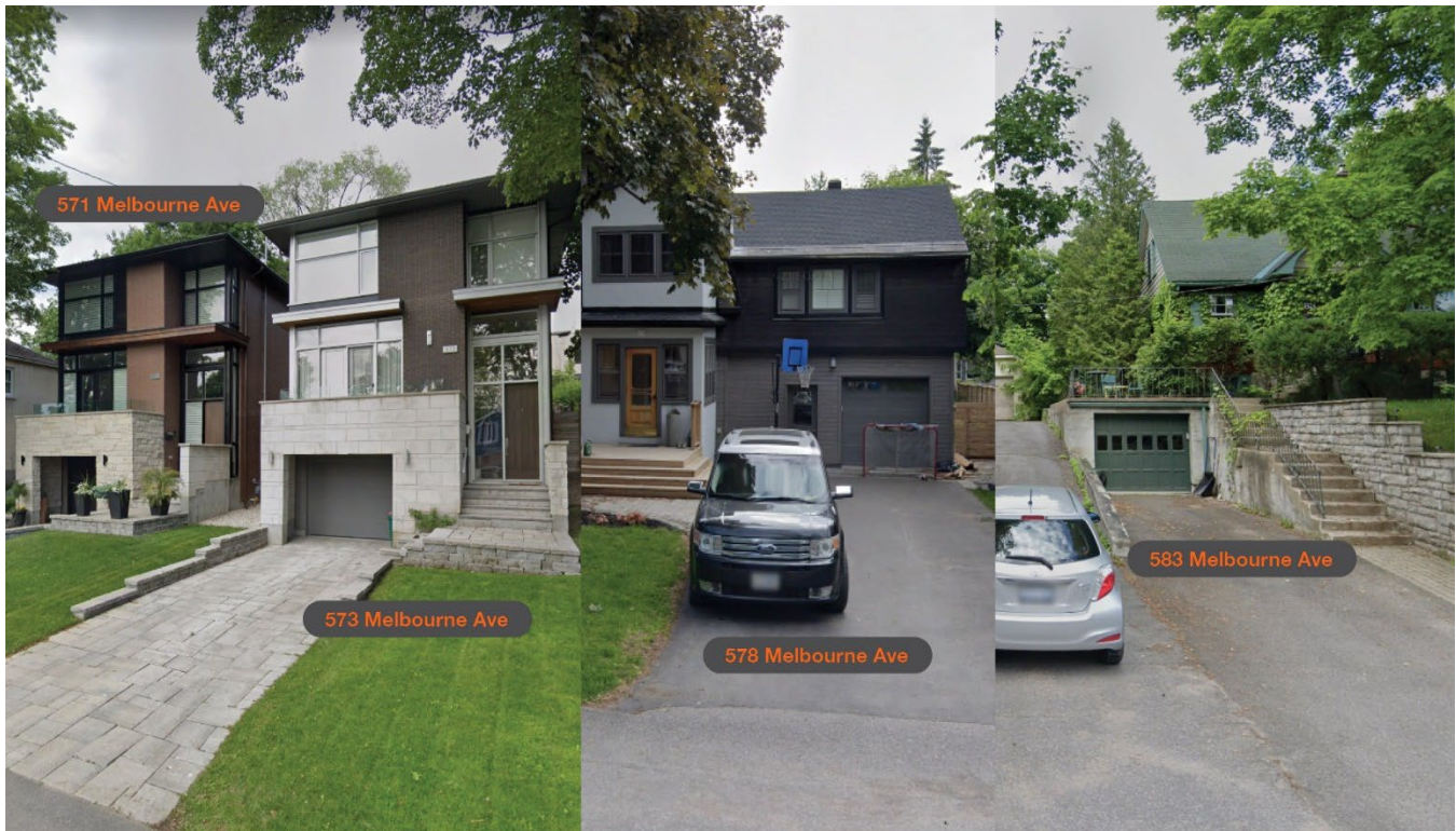
Figure 15: Existing front-yard conditions on the surrounding properties displaying the front-facing garages and driveways.
