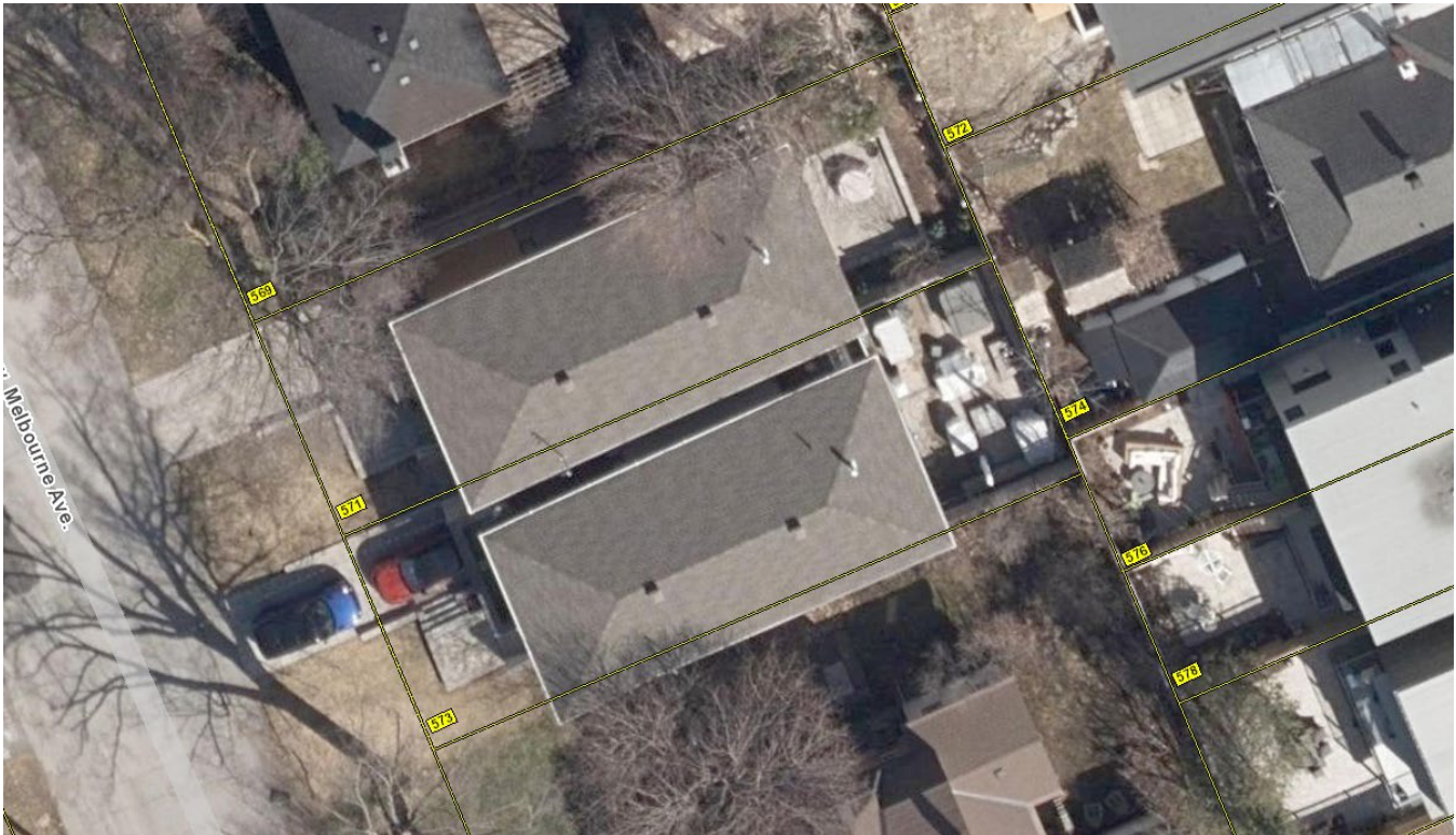
Figure 16: 573 and 571 Melbourne Avenue, depicting the similar rear-yard conditions.
