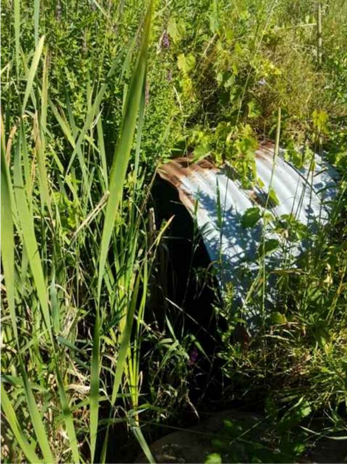
17-Culvert 1+700 - Upstream end ~1400mm CSP good condition.jpeg
