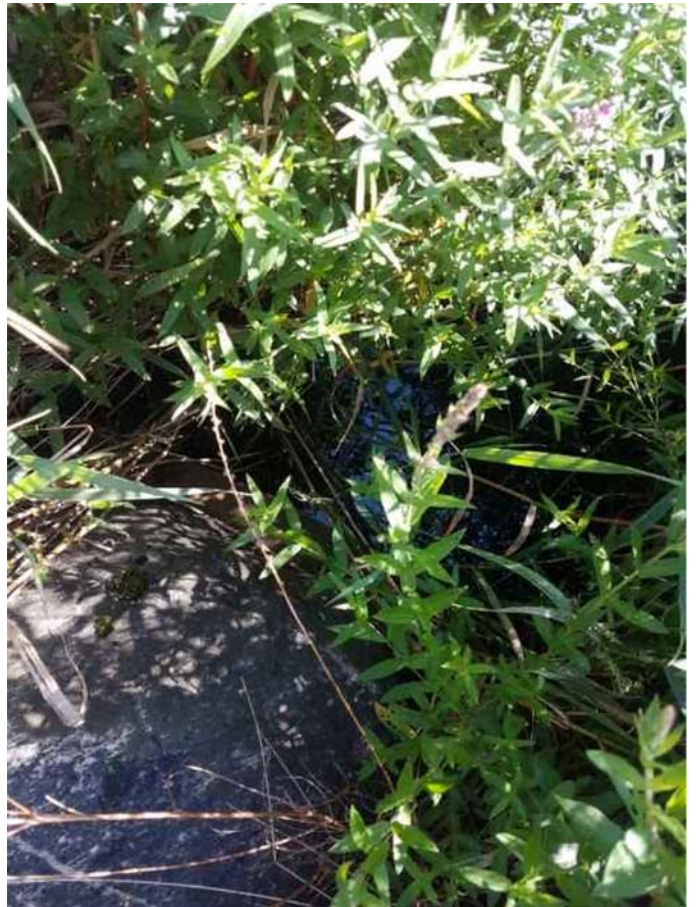
14-Culvert 1+350 - Downstream end.jpeg
