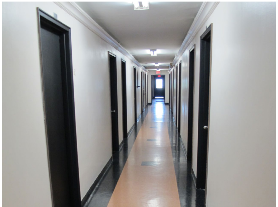
right: Interior corridor
