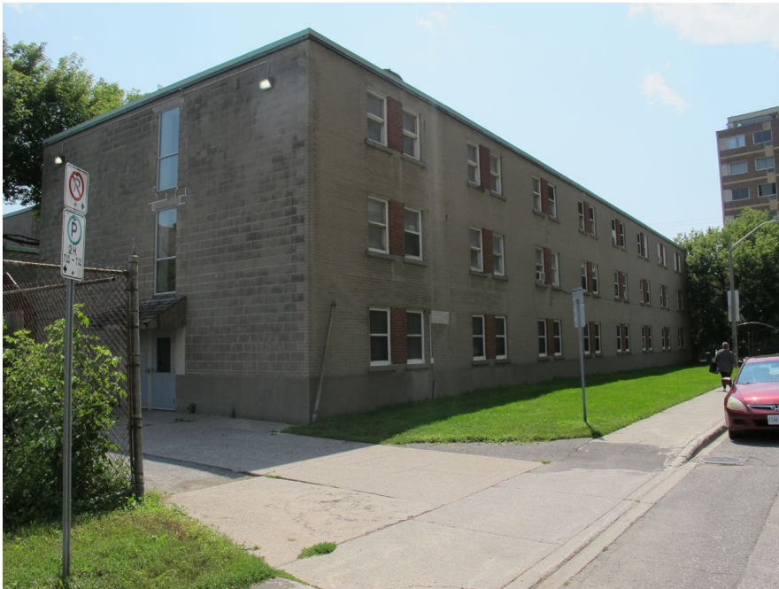
Nurse's residence wing north and east elevations
