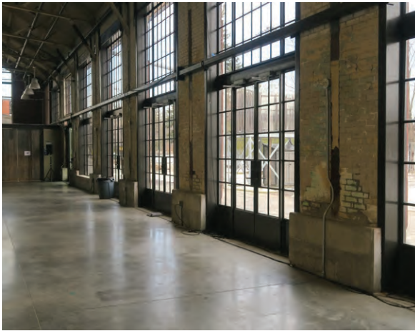
Deteriorating brick walls on the east interior elevation of the exhibition hall (ERA 2023)
