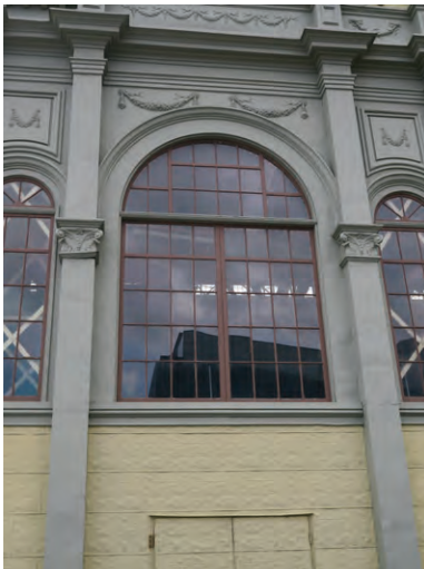
Entrance Pavilion window on north elevation (ERA 2023)
