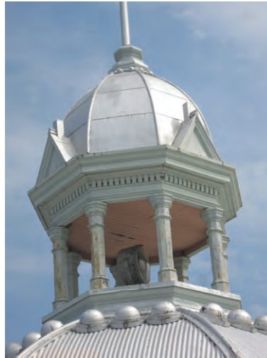
Roof cupola from south (ERA 2019)
