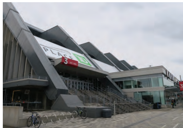
East and north (primary) elevation of TD Place (ERA, 2023).
