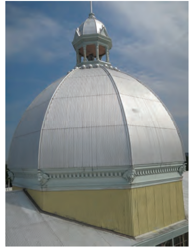
South view of roof dome (ERA 2019)
