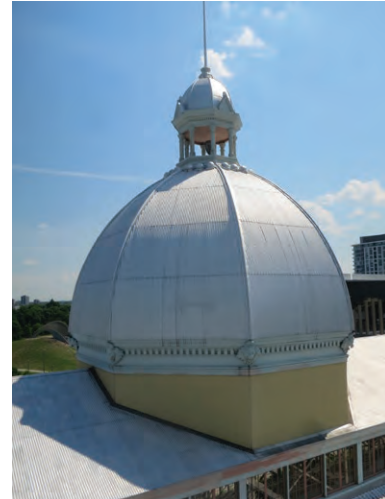
General view of roof dome from north side (ERA 2019)
