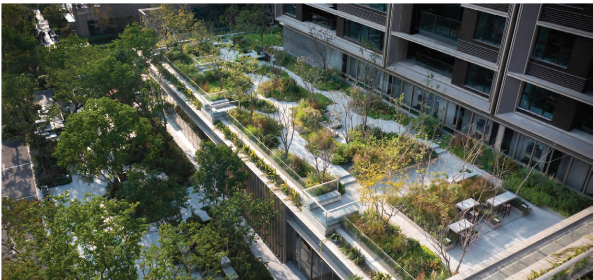
Urban Valley Commercial District TROP (Archdaily)
