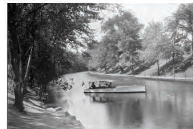
Undated photograph of Rideau Canal above Bank Street (Library and Archives Canada).
