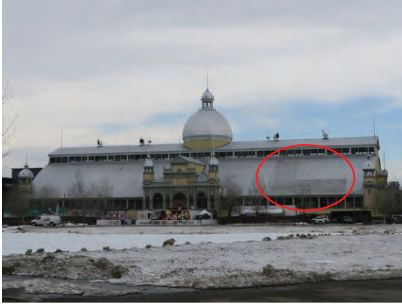
South lower roof. Note fabric covering (ERA 2023)
