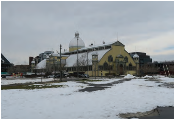
Looking northwest across the Great Lawn towards the Aberdeen Pavilion (ERA, 2023).
