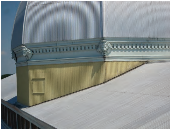
Base of roof dome from north side (ERA 2019)
