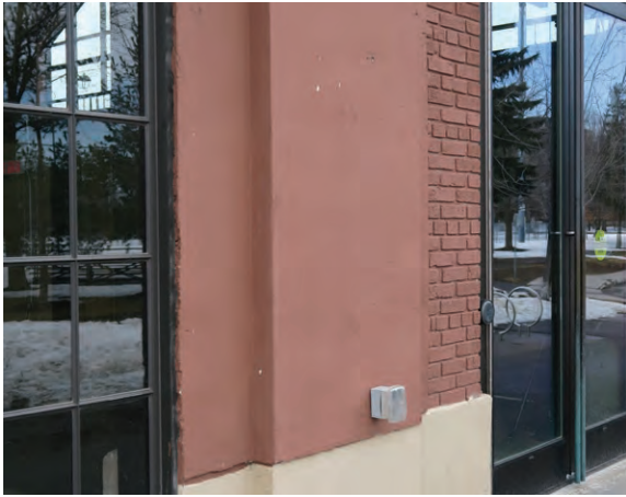
Cement render applied onto the brick on the east elevation (ERA 2023)
