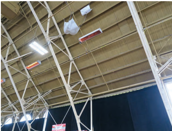
Wood roof purlins and decking. Note gaps between wood decking and rain capture tarps (ERA 2023)
