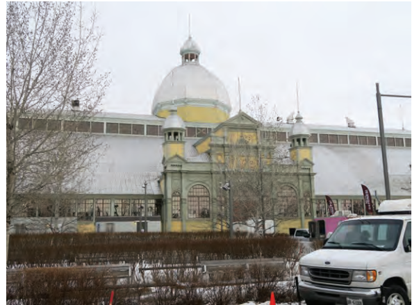
South elevation entrance pavilion (ERA 2023)
