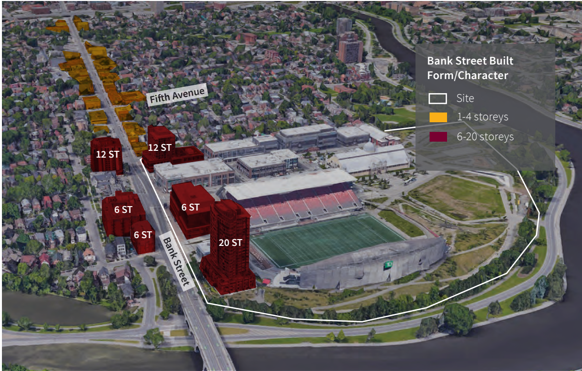
Axonometric northwest view of the Site and Bank Street (Google Earth, 2021; annotated by ERA).
