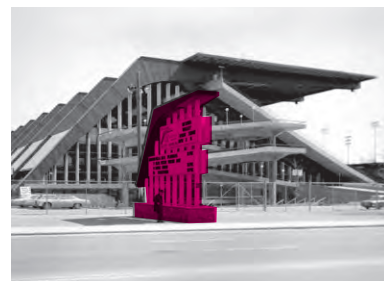
1960s signage (shown in pink) at Frank Clair Stadium and Ottawa Civic Centre (Adjeleian Allen Rubeli Limited, n.d.; annotated by ERA).
