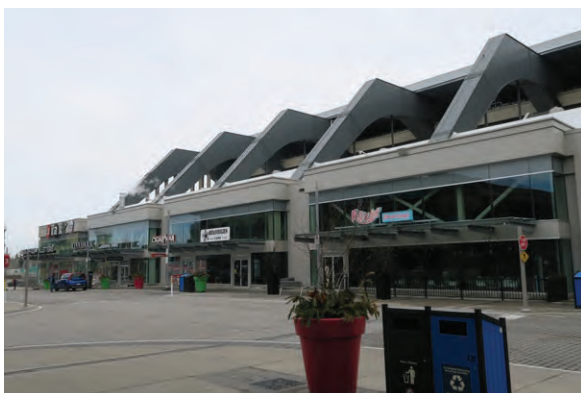
Eastern portion of the podium on the primary (north) elevation of TD Place (ERA, 2023).
