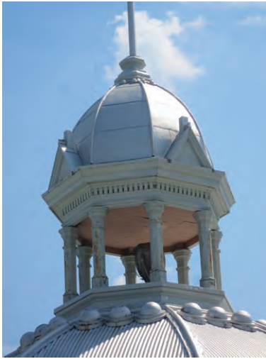
Dome roof cupola from north side (ERA 2019)
