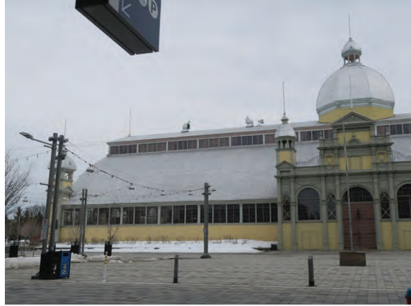
North upper roof: east section. (ERA 2023)
