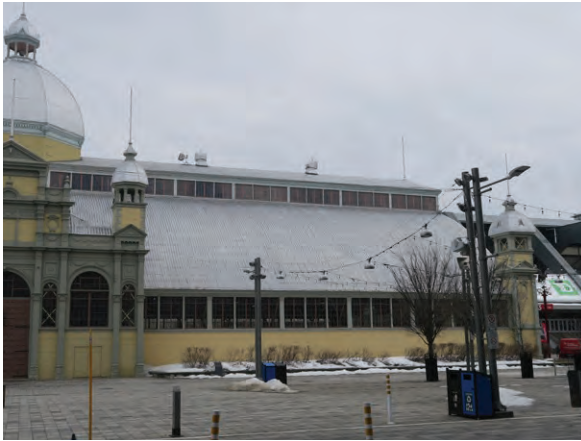
North upper roof: west section (ERA 2023)
