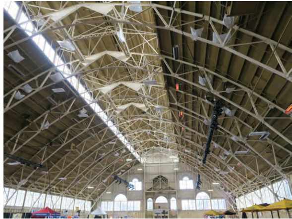
Interior underside of roof: looking west (ERA 2019)
