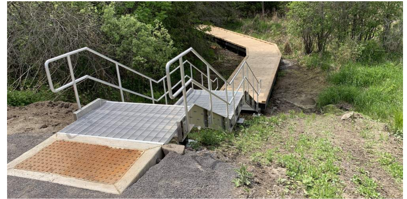
Image 1.29 Kizell Trail Expansion stair - Source: CSW
