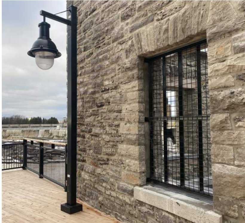
Photo 1: Black metal grilles installed at Chaudiere Falls Lookout, in Ottawa. Grilles were designed as guardrails to protect the public from a fall hazard. Spacing of metal bars mimic original window detailing.
