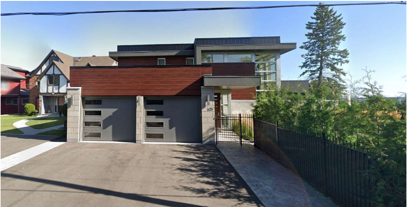
Figure 4: The neighbouring property to the west, being 123 James Cummings Ave., was developed in 2017 and has a garage set forward from the principal entrance.
