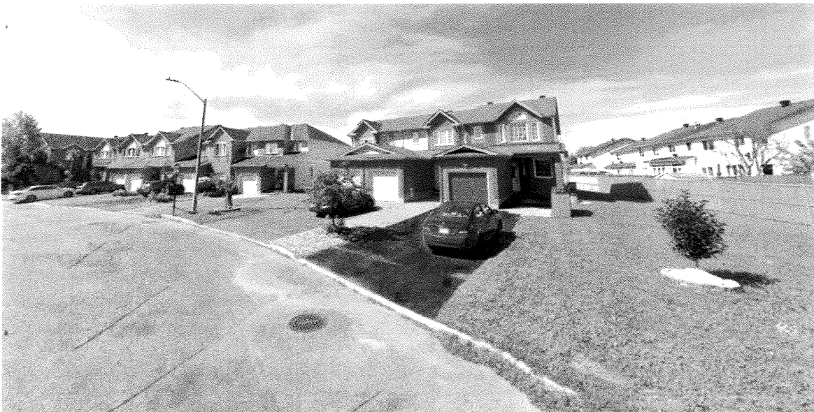
Figure 10: View along Pennard Way, looking west
